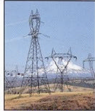
Powerlines across the region
