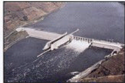
Lower Granite Dam
