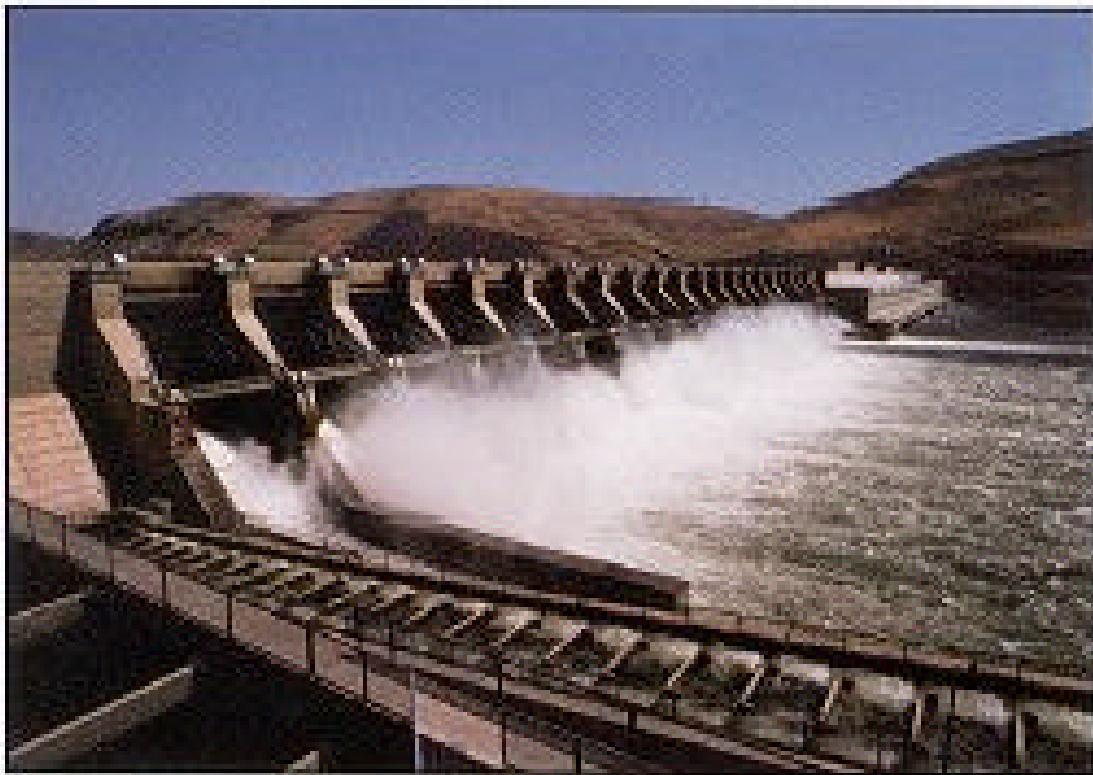
Spilling water at John Day Dam.
