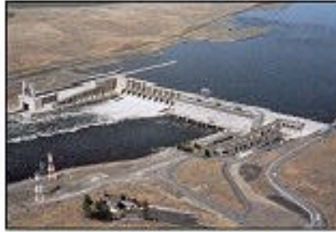
Ice Harbor Dam
