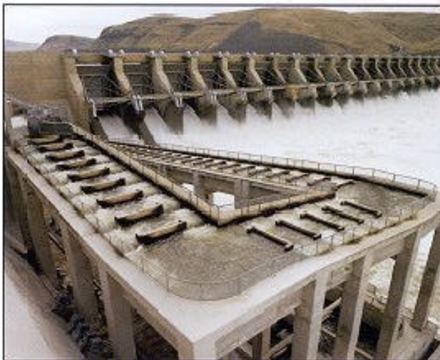
John Day Dam fish ladder system
