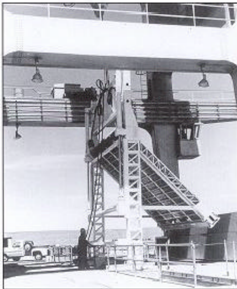
First prototype of Turbine Intake Traveling Screen, tested at Ice Harbor Dam in 1969.
