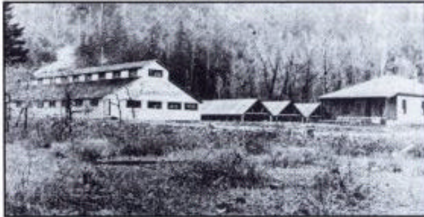
Central Salmon Hatchery, showing the incubation building (left), sheds, and a residence (right), 1910s.
