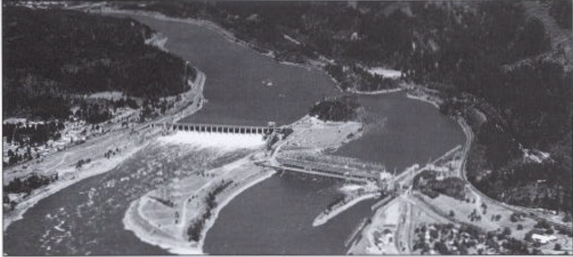
Bonneville project after completion
