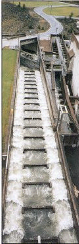
The fish ladder is a stairstep to help lift the fish to the upper pool beyond the dam.
