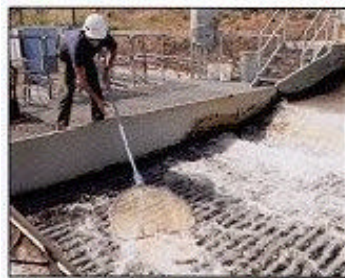
Large fish are separated from small after exiting the bypass flume
