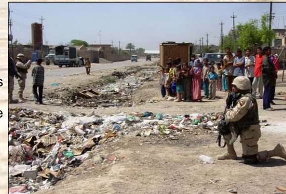
Sewer trenches in Baghdad are frequently filled with trash. — Photo by Steve Purdy
