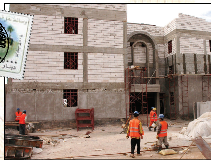
New courthouse takes shape.
