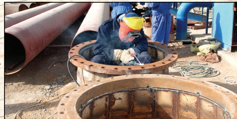
Iraqi crew is quadrupling size of Basra water treatment facility.
