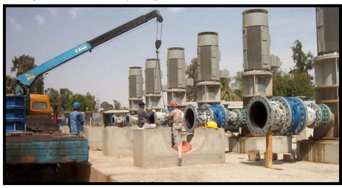
Here is an inspection of a water supply project of ours. The workers will connect the pumps shown to a large header. This photo on the right is of me during my duty of escorting local nationals to our USACE, Kirkuk Area Office for business.
