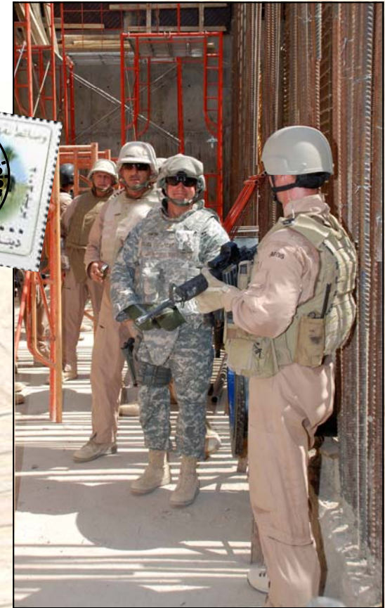
Progress at Fallujah's first ever sewer system project
