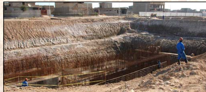
Wastewater Pump Station foundation work
