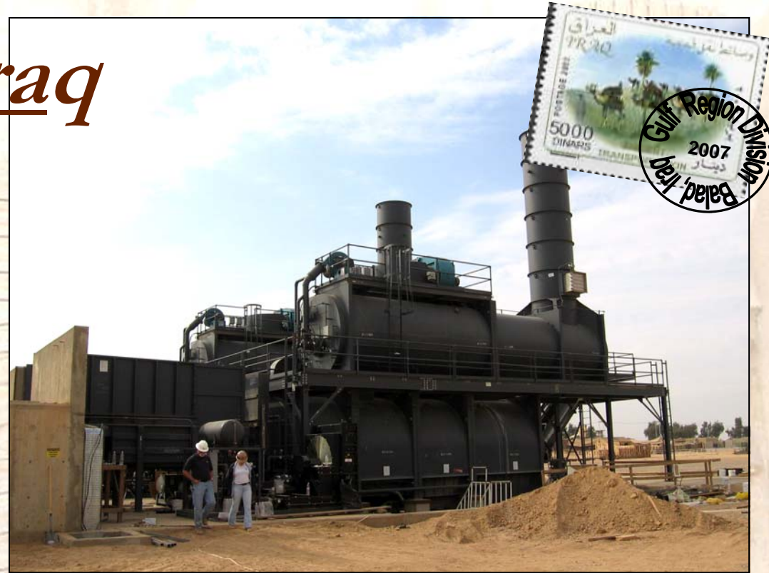
Anaconda Incinerator Units 1 & 2—This Military Construction project is one piece of a solid waste management plan for LSA Anaconda. Once the plan is fully implemented, it will provide a means of disposal of camp trash that is now being burned in an open pit. This will greatly enhance the health and quality of life for the Anaconda residents as well as the nearby villages. GRN file photo.
