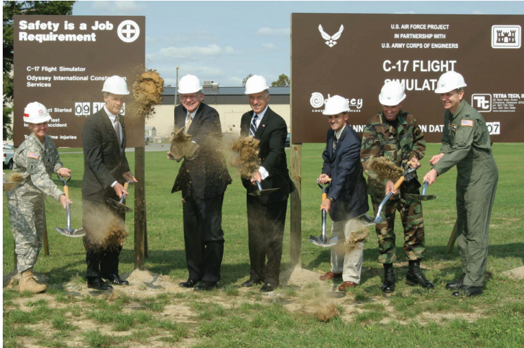
(From left) Lt. Col. Gwen Baker, Sen. Tom Carper, Rep. Mike Castle, Sen. Joe Biden, Dover Mayor Stephen Speed, and Air Force Cols. Sam Cox and David Wuest toss the proverbial first dirt during the Sept. 11 groundbreaking at Dover Air Force Base for a new C-17 simulator facility. The ground breaking made way for the C-17 Globemaster III flight simulator and flightcrew training facility. The C-17 will complement the base's current fleet of C-5s by providing a new, modern capability in line with the varying Air Mobility Command's missions of the 21st century.
