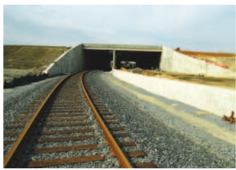
RUNWAY CONSTRUCTION AT THE PHILADELPHIA INTERNATIONAL AIRPORT
