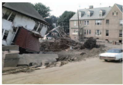
PROPERTY DAMAGE CAUSED BY TROPICAL STORM AGNES
