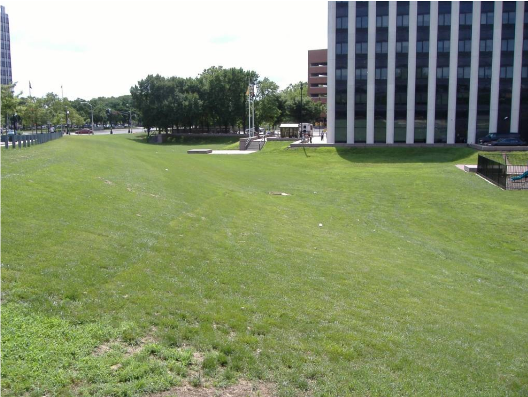
Plate 2. View downstream of turf and fill covering the Broad Street culvert.
