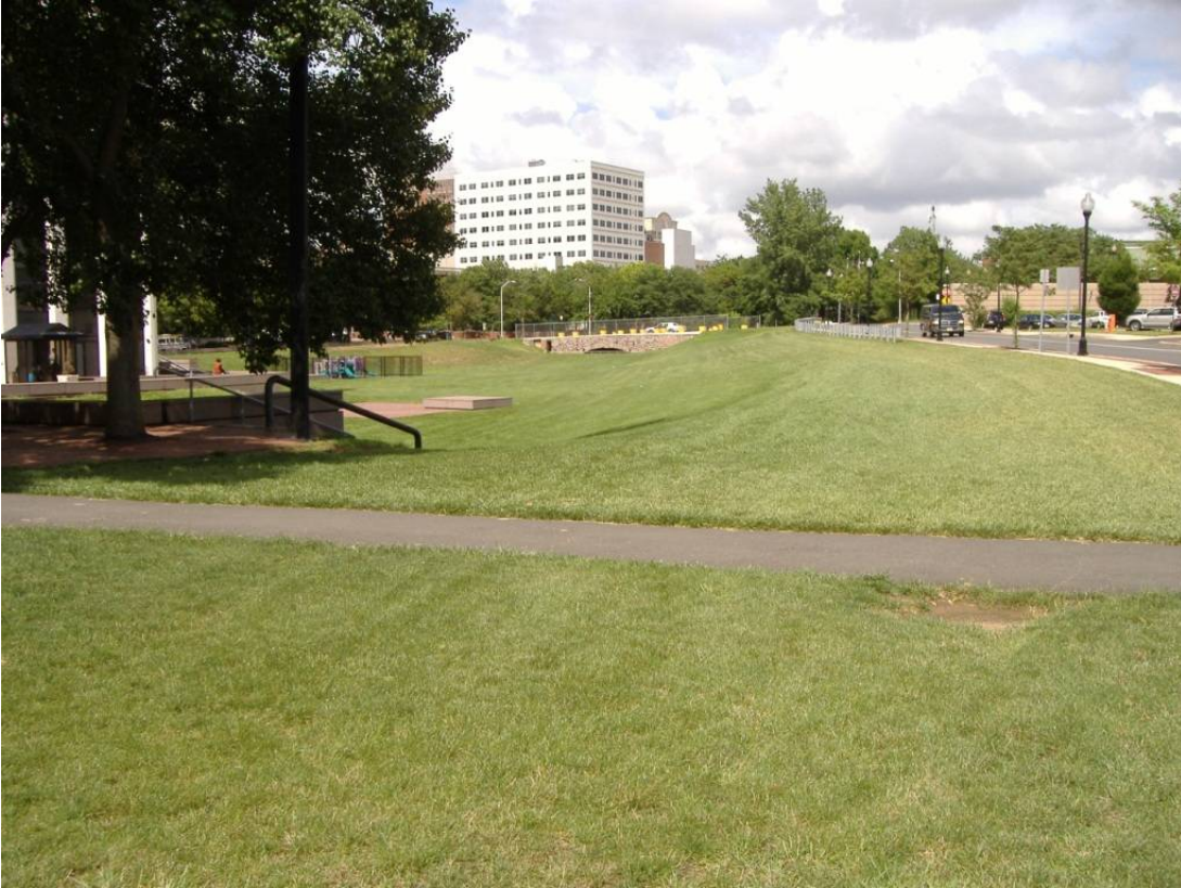
Plate 1. View upstream of turf and fill covering the Broad Street culvert.
