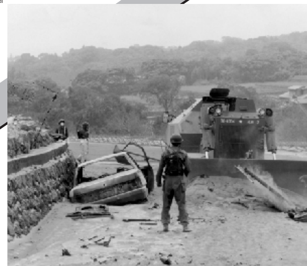
SDF members restoring road damaged by large-scale pyroclastic flow at Unzen-Fugendake by removing sizzling volcanic ash with use of 75-type bulldozer; four bodies are found in vehicle shown left (Nagasaki Prefecture on June 5, 1991)
