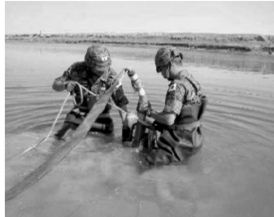
SDF members installing sluice gate for water supply (March 2004)
