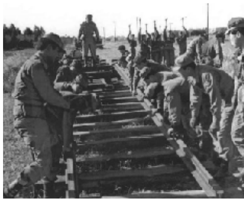
Members of SDF's 101st construction unit demonstrating laying of railway track (training site in Tsudanuma in Chiba Prefecture in June 1960)
