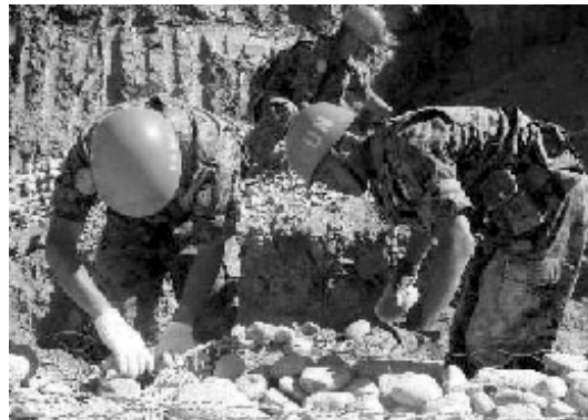
SDF members engaging in road restoration work (June 2002)
