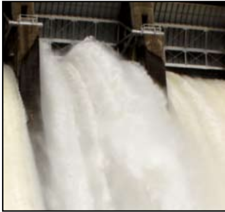
Norfolk Dam Spillway
