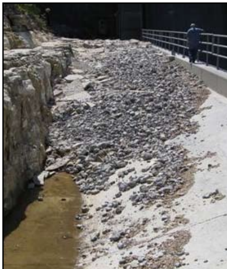
Beaver Dam Retaining Wall
