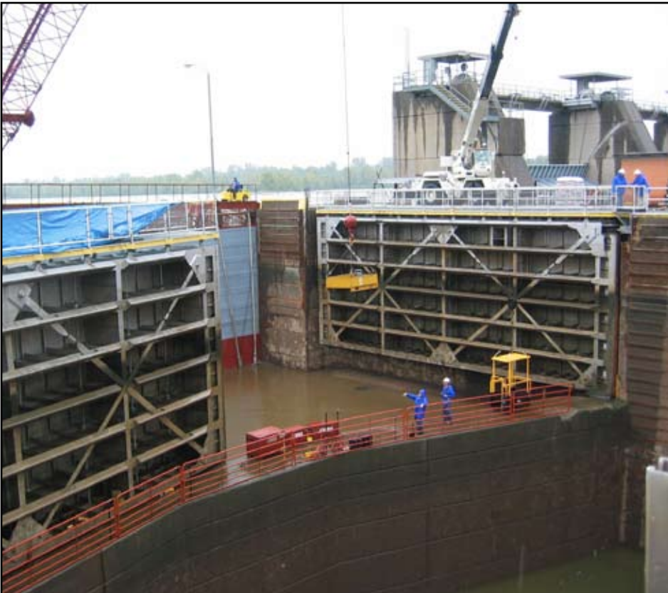
Dewatered Lock Chamber
