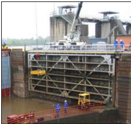
Dewatered Lock Chamber
