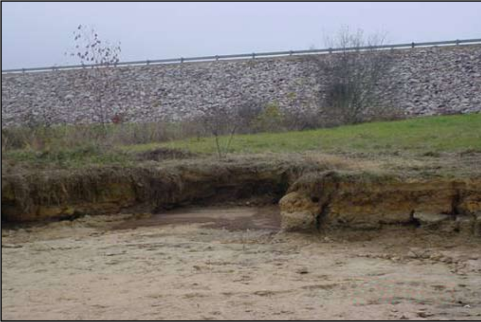
Millwood Dam Embankment
