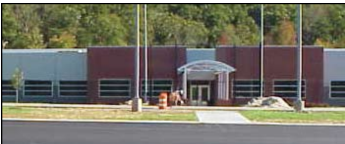
DOE Agent Facility
