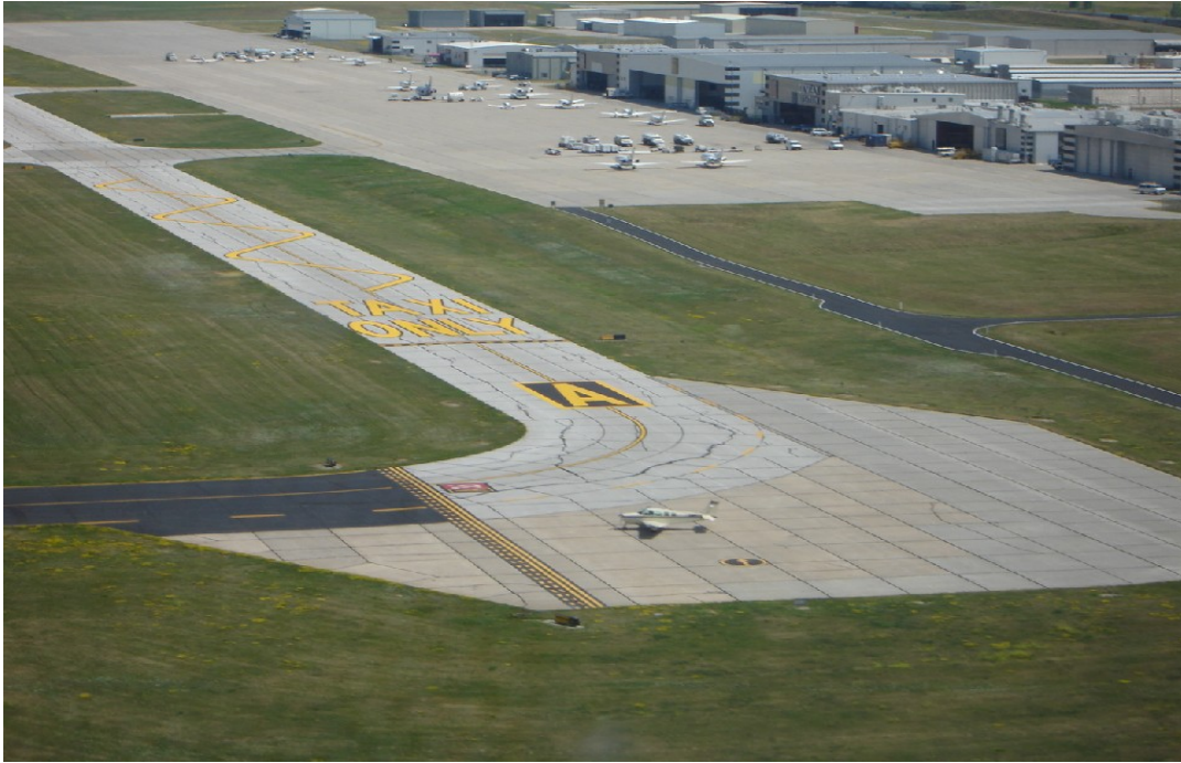
Figure A-13. Nonstandard Paint Markings on Taxiway Alpha at Lincoln Airport (LNK)
