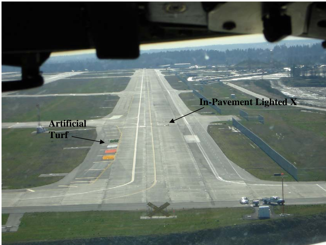
Figure A-21. In-Pavement Lighted X in Operation With Artificial Turf on the Left Shoulder of Taxiway Tango (SEA-TAC)
