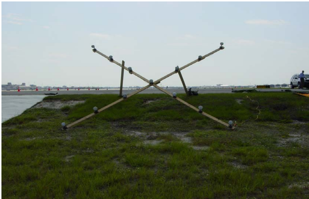
Figure A-23. Temporary Elevated Lighted X in Water Retention Ditch (PBI)
