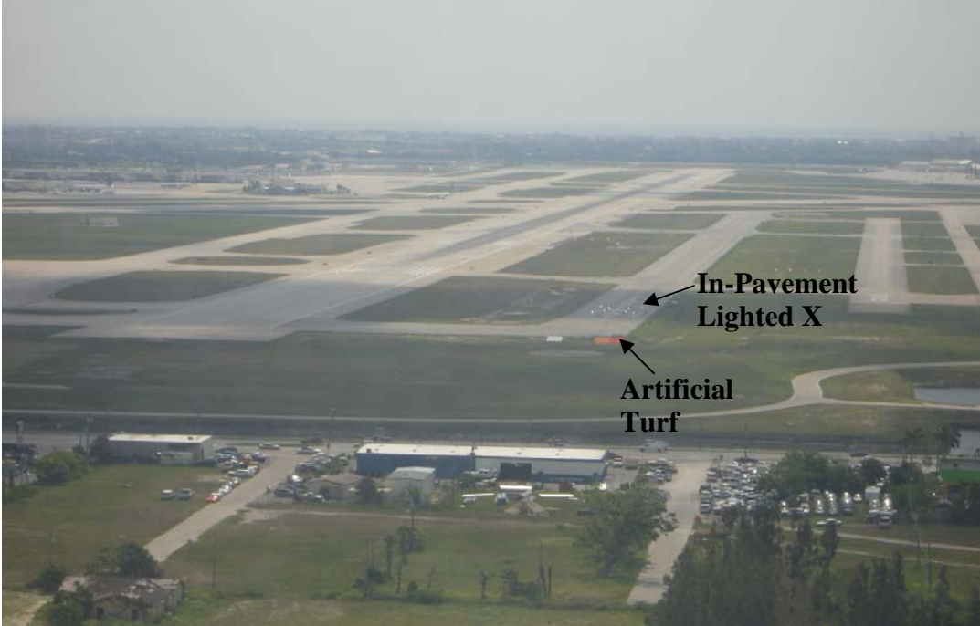
Figure A-26. In-Pavement Lighted X Illuminated on Taxiway Lima (PBI)
