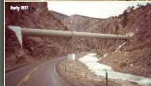
Sample view of the Big Thompson River channel at the mouth of the river. The debris dam is the result of the flood. The debris dam is the result of the flood.
