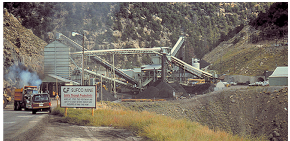
Figure 7C. The SUFCO mine, owned by Canyon Fuel Company, operates in Convulsion Canyon in the Manti-La Sal National Forest, southern Wasatch Plateau, Utah. Photo by R. Dubiel, U.S. Geological Survey.
