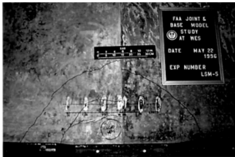
FIGURE 7-42. POSTTEST PHOTOGRAPH OF TOP SURFACE OF SLABS, EXPERIMENT LSM-5
