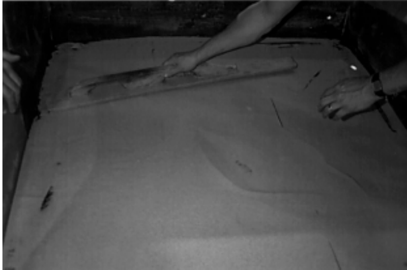
FIGURE 7-9. PLACEMENT OF THIN SAND LAYER
