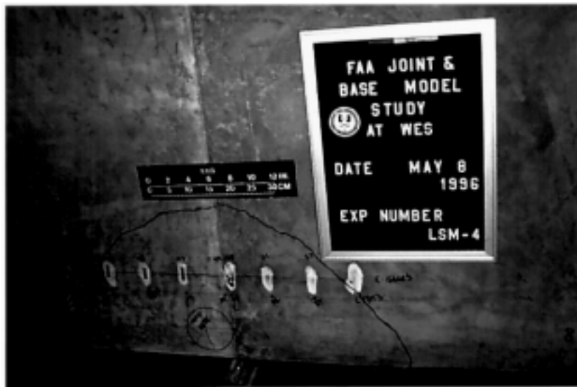
FIGURE 7-38. POSTTEST PHOTOGRAPH OF TOP SURFACE OF SLABS, EXPERIMENT LSM-4
