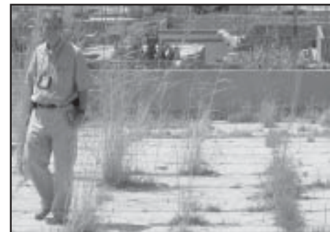
Jim Peak inspects the leaky roof of a school in Dahuk, Iraq.
