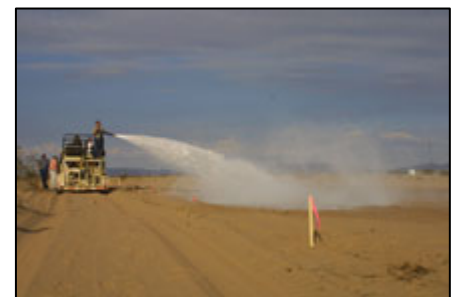
ERDC researchers use a hydroseeder to create a dust-free helicopter landing pad in Yuma, AZ
