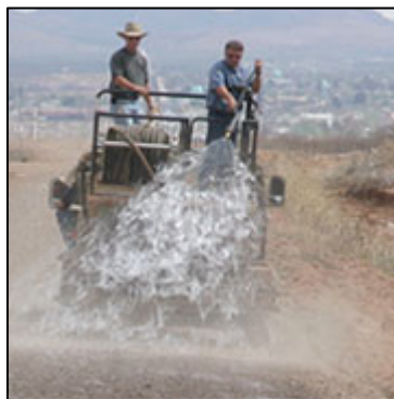
Dust mitigation on a U.S. Border Patrol road, using trailer-mounted hydroseeder pulled by a HMMW
