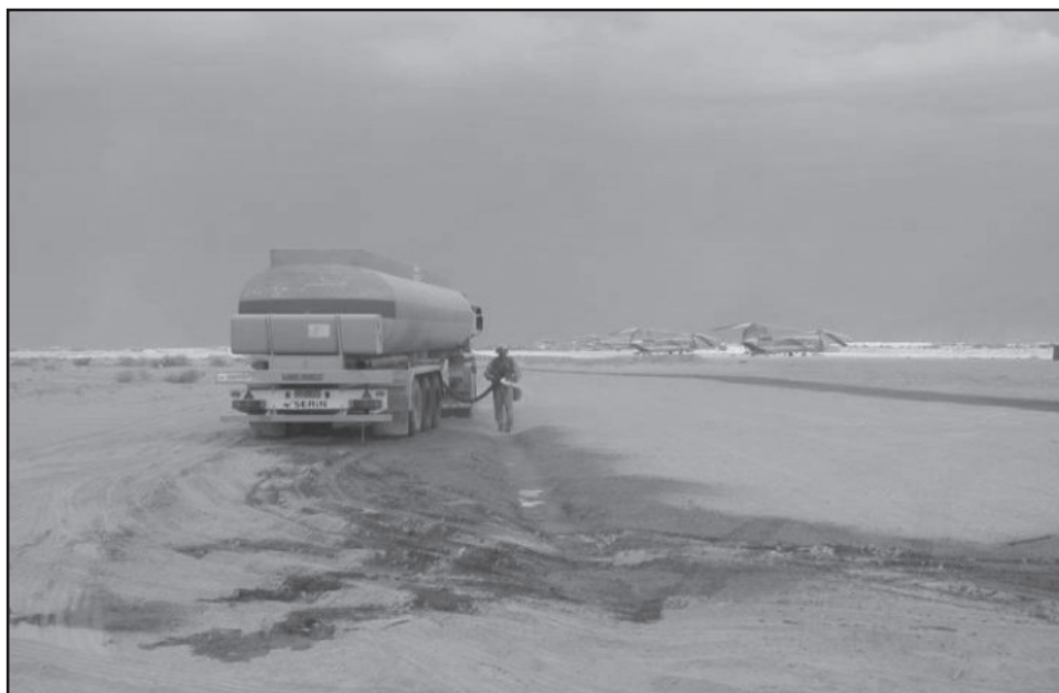
Figure 101. Using oil for dust abatement at FARP SHELL
