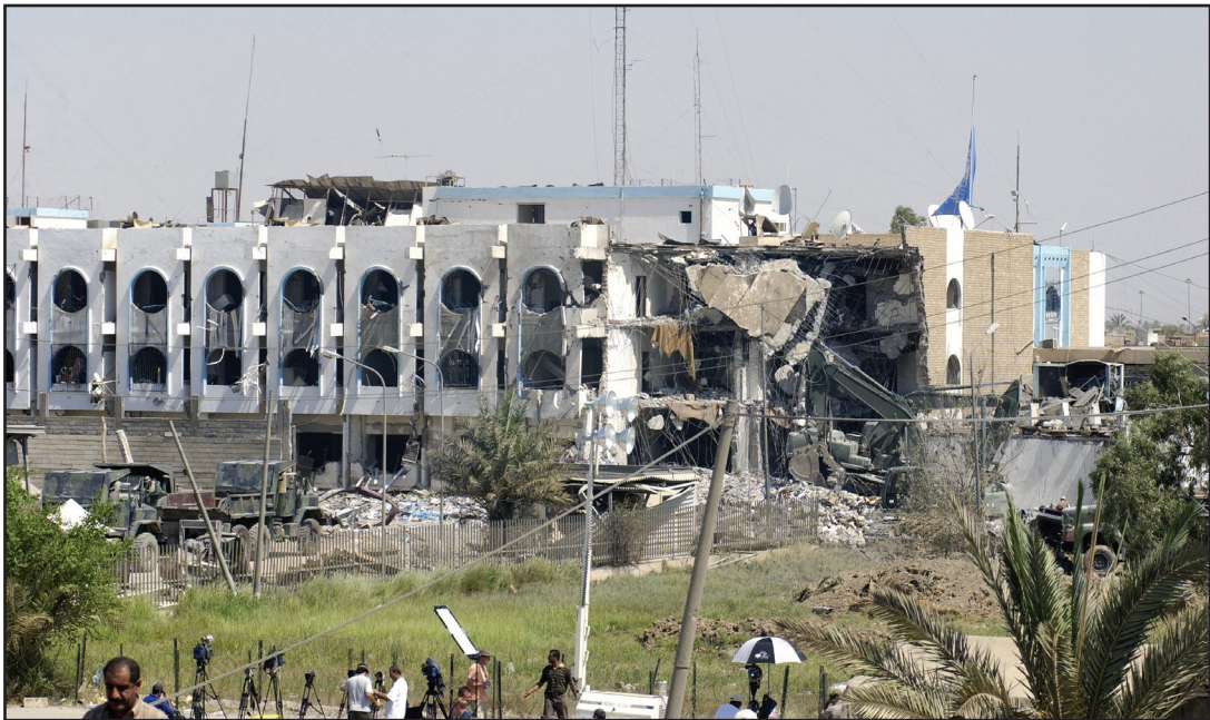
Figure 16. Long shot wide-angle view showing damage to the UN Headquarters building in Baghdad, Iraq, following a truck bombing that destroyed a portion of the building.
