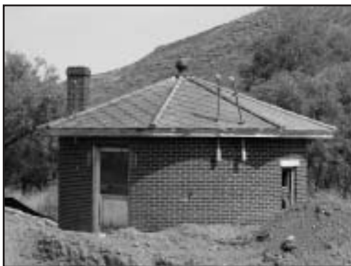
The historic roundhouse from Fort Benton's water treatment plant will serve as the pump house at the new Upper Missouri River Breaks National Monument Interpretive Center. Photo by Zane Fulbright
