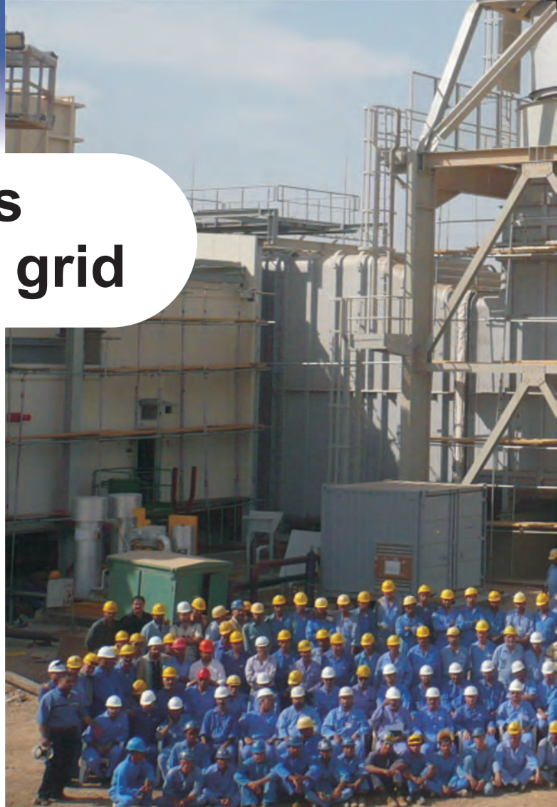
The $170 million Qudas Generation Plant expansion features two huge General Electric Frame 9E generators that will add much needed megawatt capacity to the grid.
