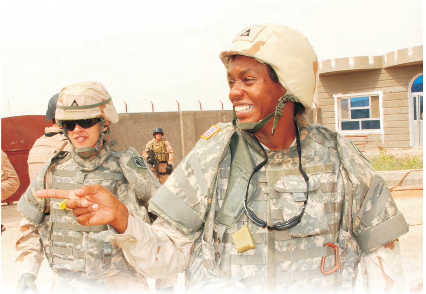
USACE Project Engineer Colleen Hickey (left) and Construction Representative Toni Graves view construction progress at the new 200-cubic-meter-per-hour facility providing additional water treatment capacity for the community.
