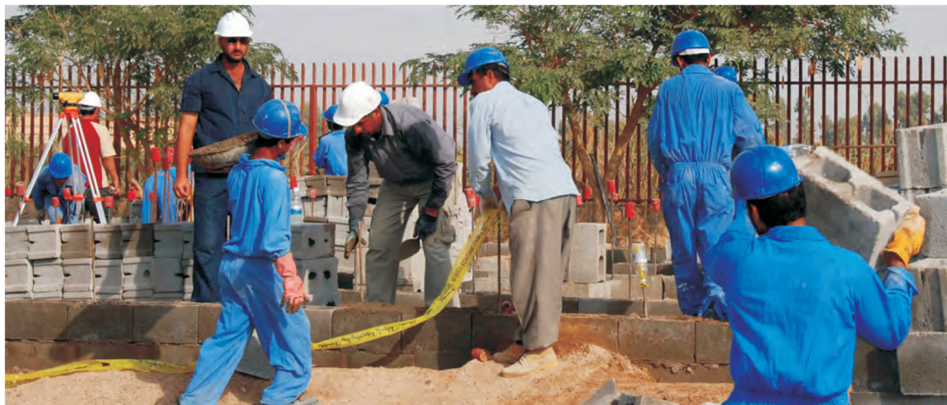
Work progresses in laying foundations for the judicial housing areas.
