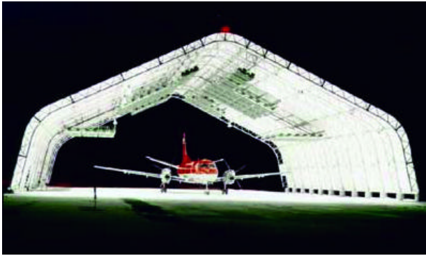
Infrared deicing facility
