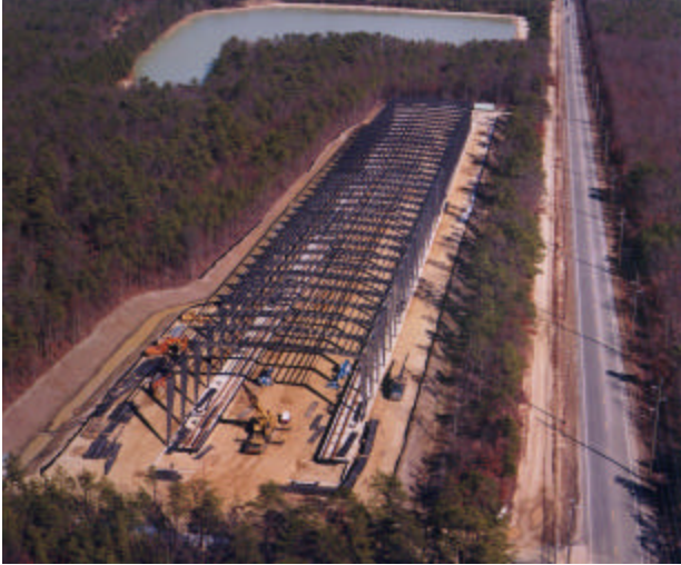
Aerial view of National Airport Pavement Test Facility under construction.
