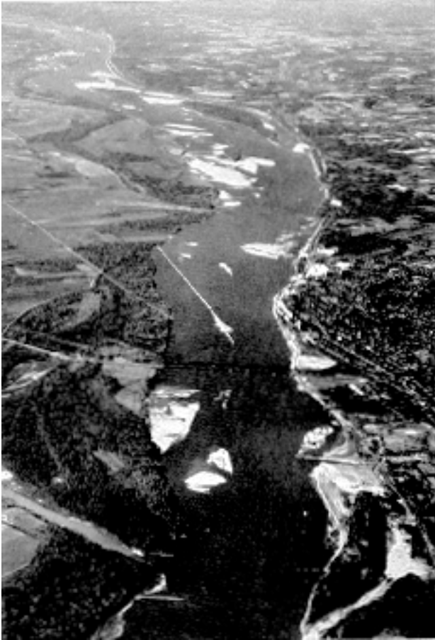
Site of Lock and Dam #26 Alton prior to construction.
