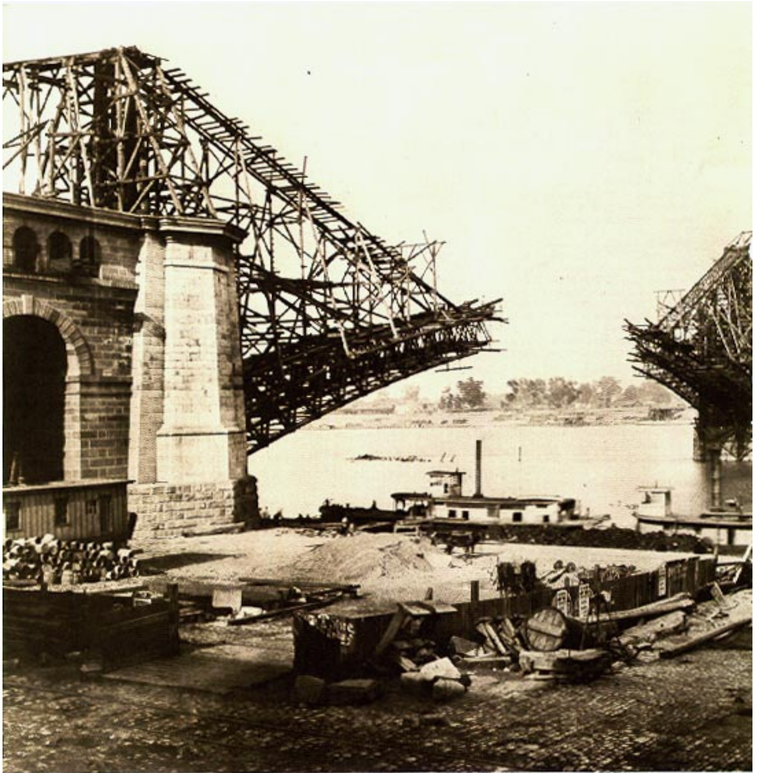
The Eads Bridge under construction.
