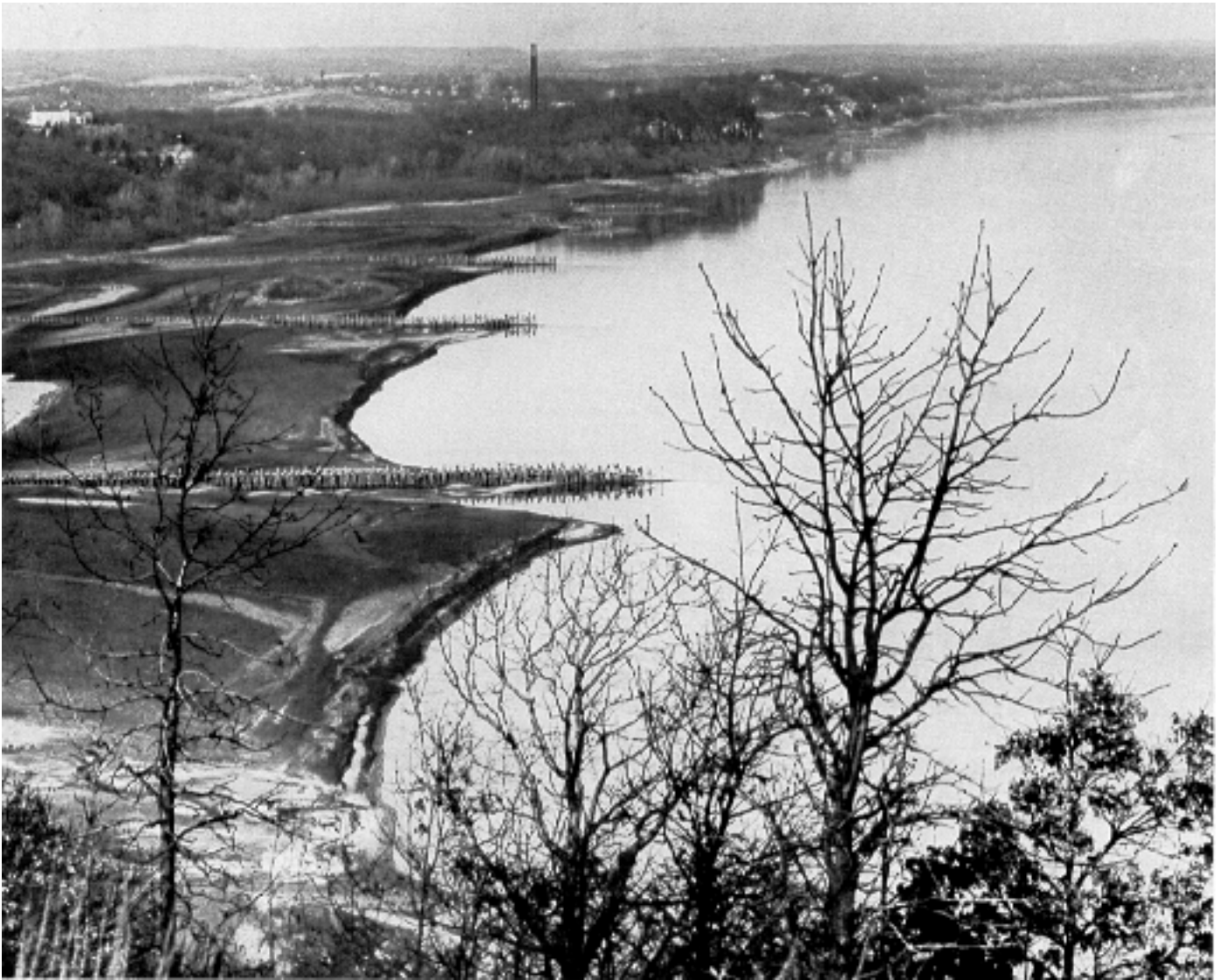
Dikes that function properly, causing accretion of sand and restricting the channel of the river. Herculaneum, Missouri, is in the background.
