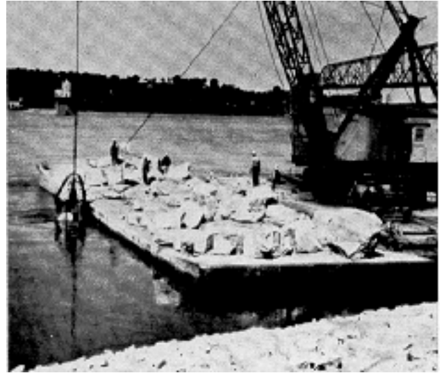
Placing rocks for Dam #27.
