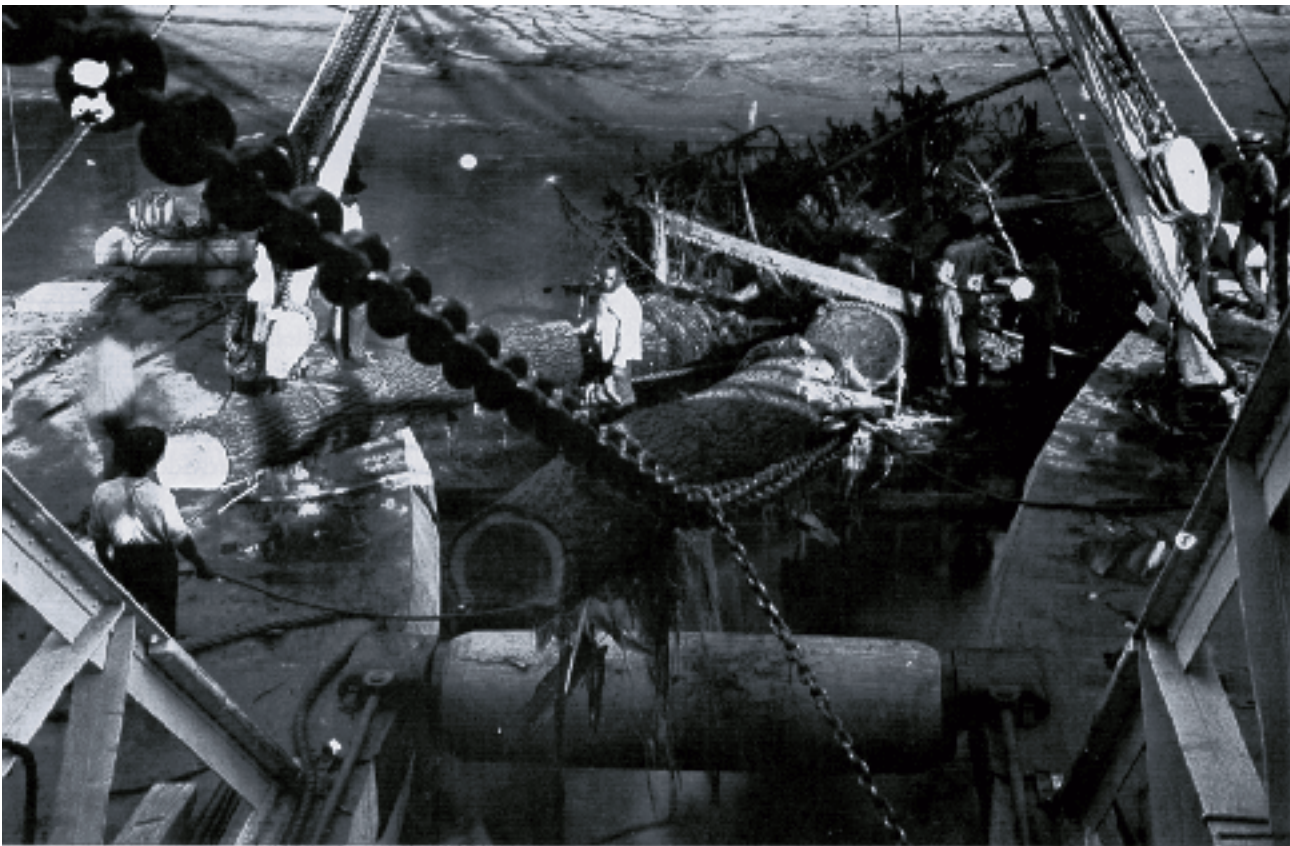
Twin snags drawn onto the butting beam of a snagboat for sawing.
