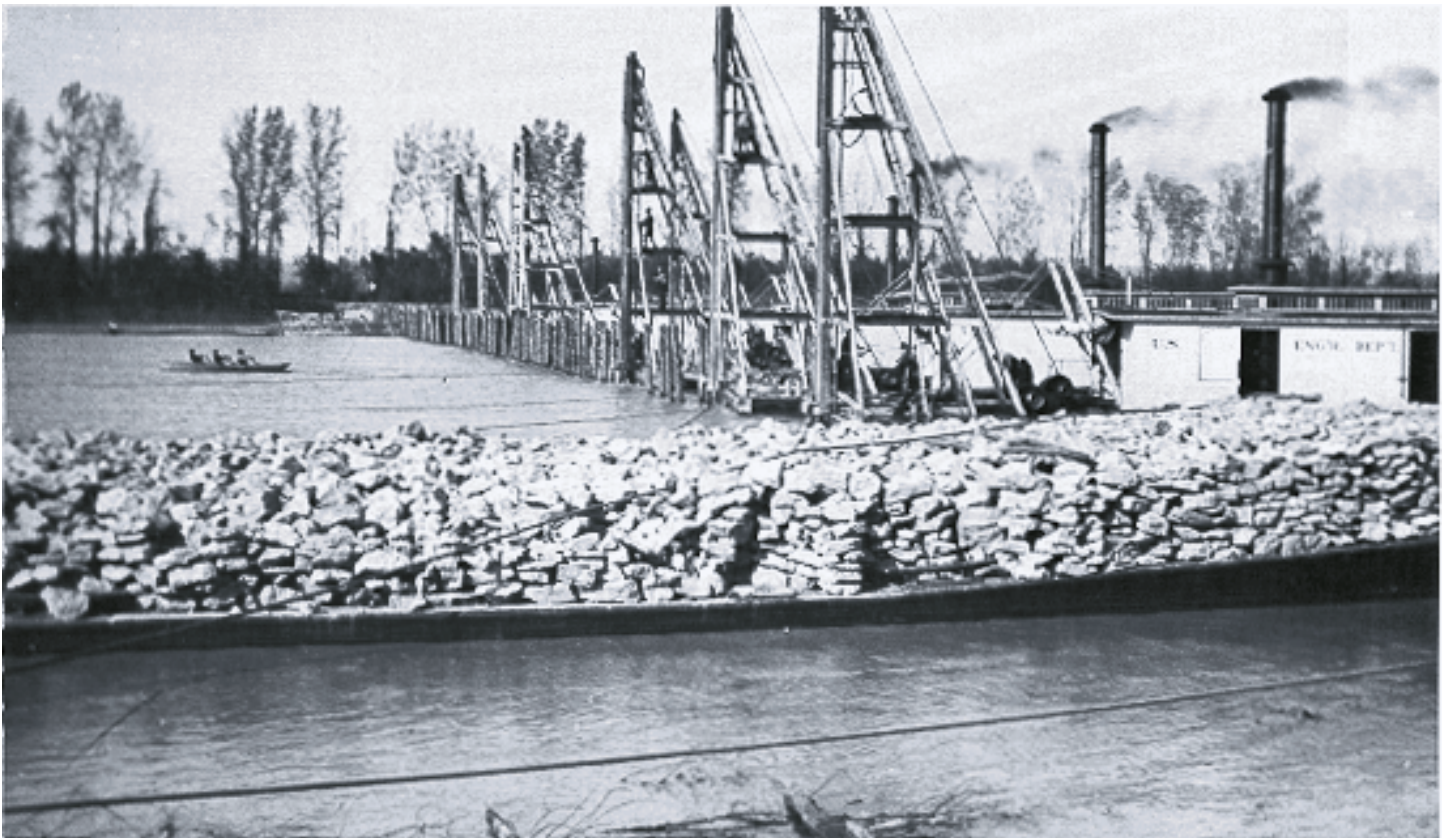
Piling dike or hurdle being constructed.
