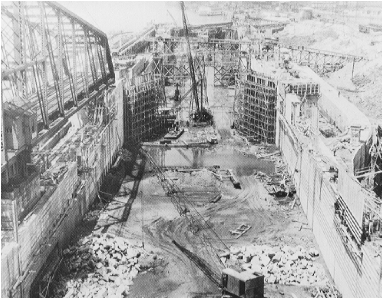
Lock #26 under construction.
