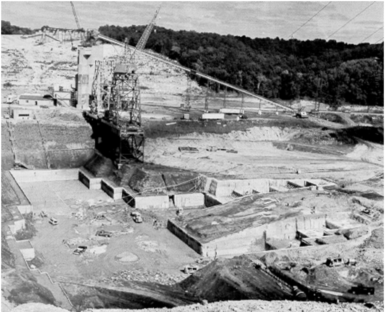
Construction of the Clarence Canyon Dam.
