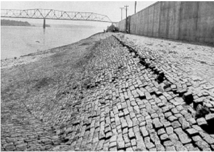
The completed Cape Girardeau floodwall.
