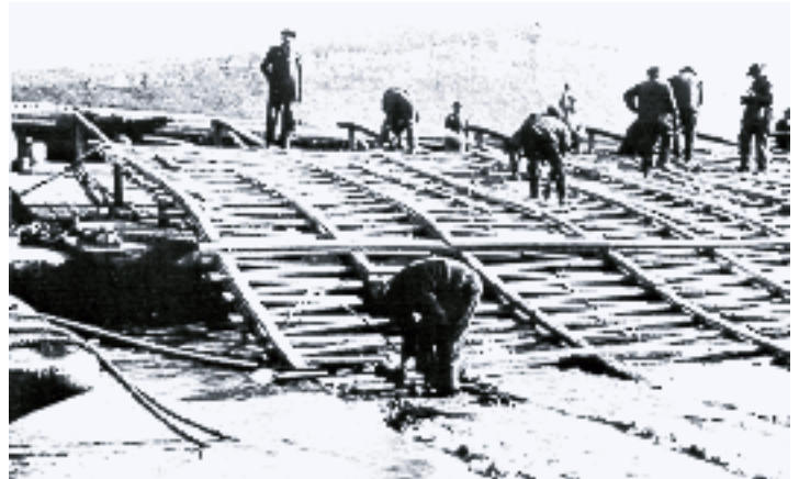
Engineer employees laying a lumber mattress revetment.
