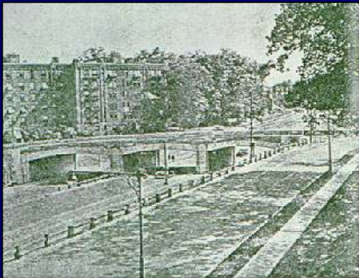
The Henry Hudson Parkway continues the West Side Highway in New York City northward to a junction with the Westchester County Parkway System, and with these connections provides a continuous express highway through the Nation's greatest metropolis. In this view the Parkway is at the left. The road at the right is one of the local service roads.
