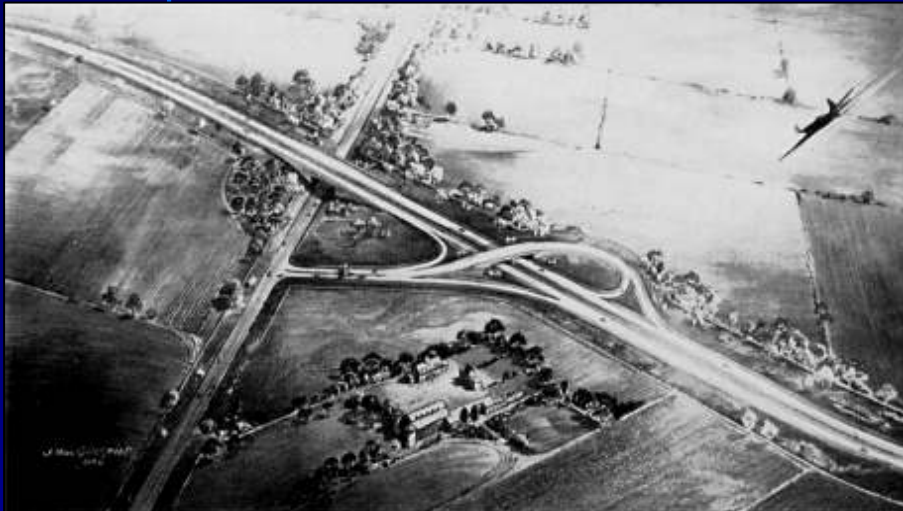
PLATE 33.—A two-lane toll road widened to four lanes approaching an access point at which only one toll booth is provided, showing the grade separating structure necessary to avoid hazards of left turns on the toll road.
