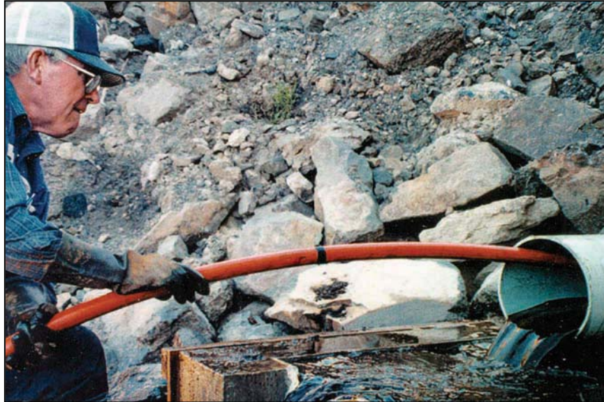
Figure 100. —Operator water jetting a drainpipe.
