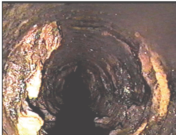
Figure 97. —Calcite deposits have formed at joints and perforations in this HDPE drainpipe.
