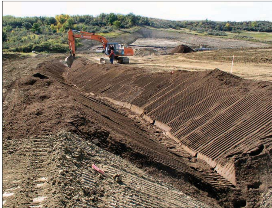
Figure 77.—Initial filter placement in a trapezoidal trench.
