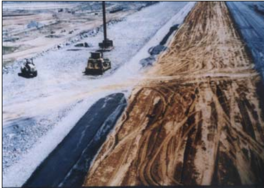
Figure 84. —Roadway crossing over a filter. Photo courtesy of ASDSO (Hammer, 2003).
