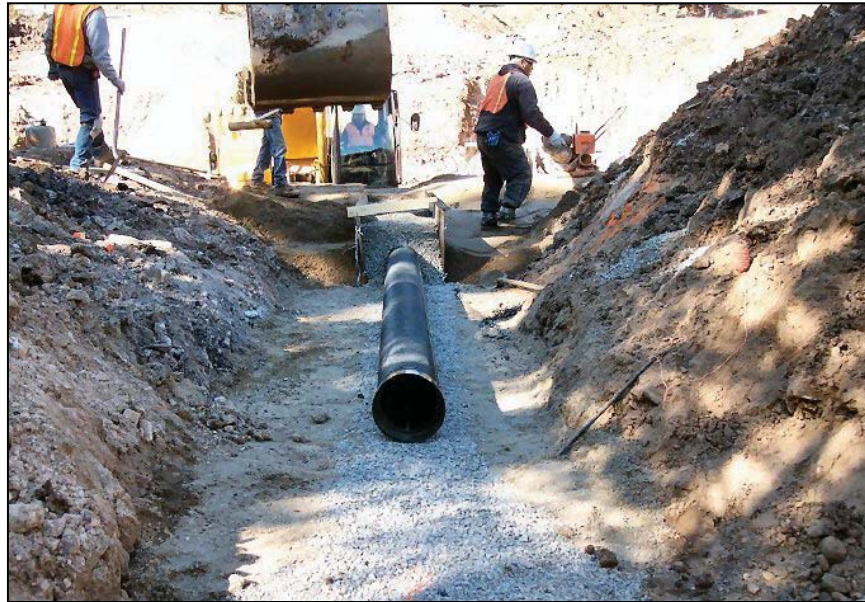
Figure 67. —Trapezoidal side slopes used in drainpipe construction.
