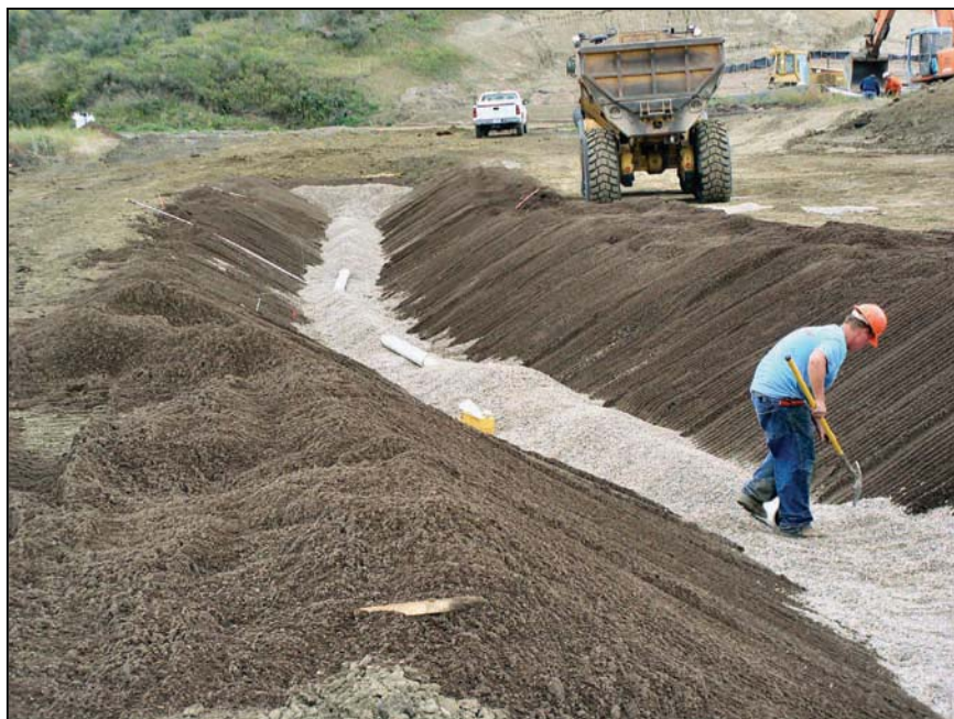
Figure 78.—Drain material being placed over a drainpipe.
