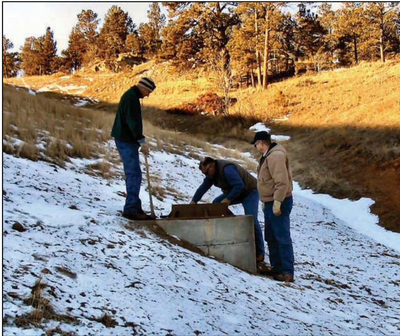
Figure 89. —Inspection well provides access to the drainpipe for CCTV inspection.
