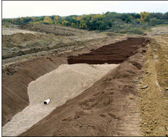
Figure 79. —Filter material being placed over drain material.
