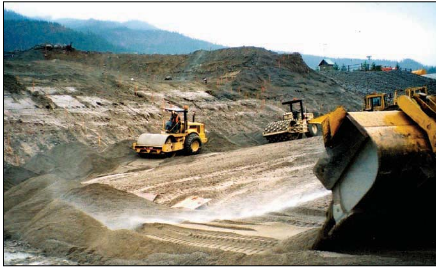
Figure 82. —Water being added to filter immediately preceding compaction. Note that this placement is occurring during a heavy rain, and wetting of the filter must continue.
