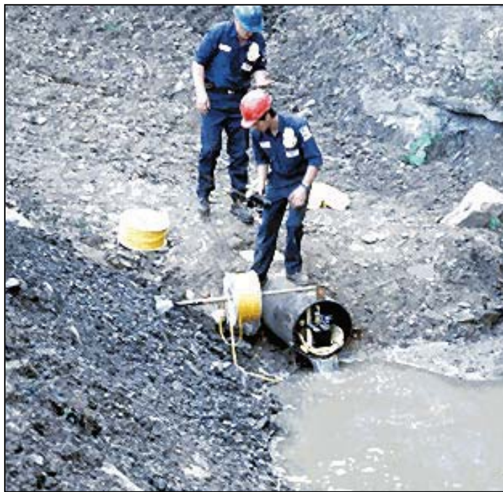
Figure 102.—Deflection monitoring of a decant pipe.
