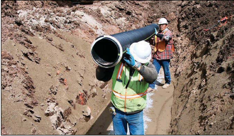
Figure 1.—Plastic pipe is lightweight, which facilitates installation.
