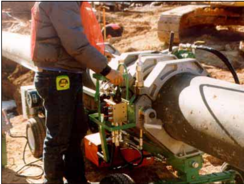
Figure 9. —HDPE pipe joint being butt fusion welded.
