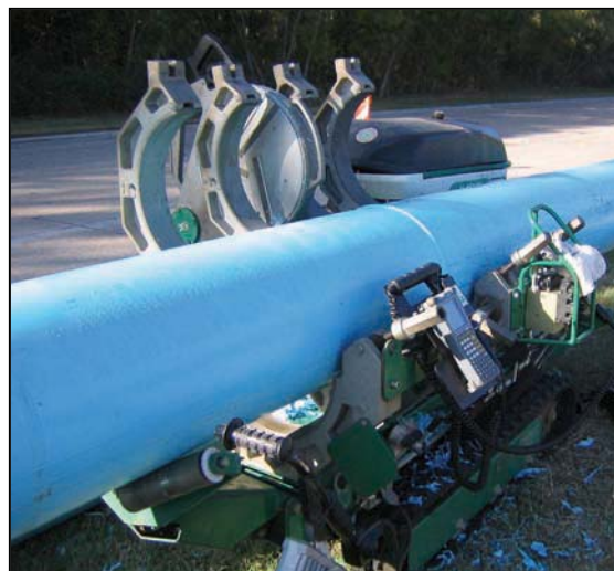
Figure 18. —The heat fusion process is used to join PVC pipe, resulting in a continuous length of pipe. Photo courtesy of Uni-Bell PVC Pipe Association Members and Associate Members.
