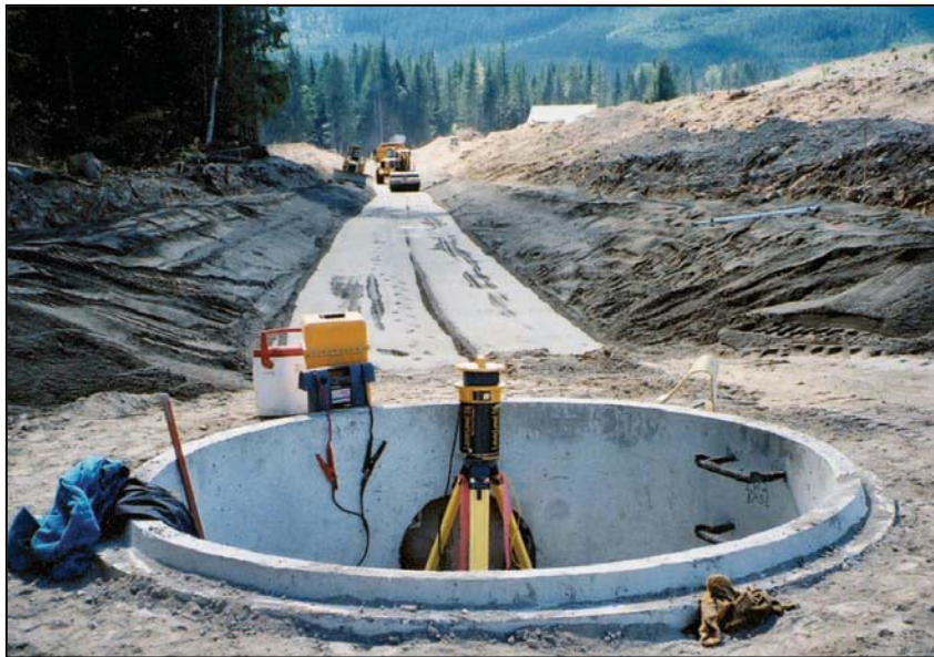
Figure 58.—The first ring of a drainpipe inspection well.
