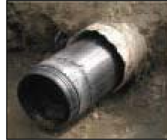
Figure 13. —Male end of snap joint.
