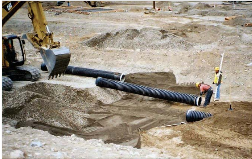
Figure 53. —Installation of profile wall corrugated pipe for a drainpipe replacement during a modification of an embankment dam.
