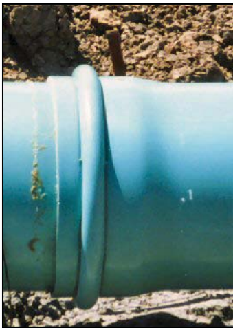
Figure 16. —PVC pipe joint (bell and spigot).
