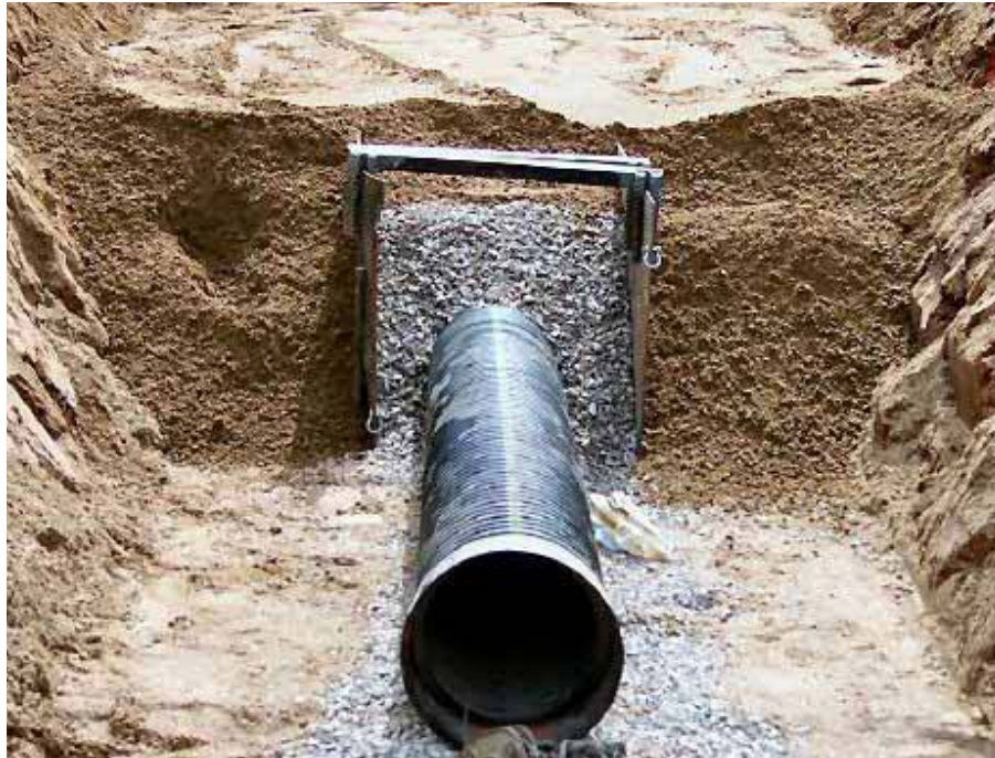
Figure 24. —A toe drain being constructed using profile wall corrugated HDPE pipe.
