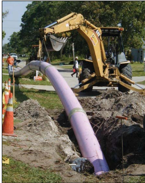
Figure 17. —The splined joint has a machined groove in the PVC pipe and in the coupling to allow insertion of a flexible thermoplastic spline that provides a 360-degree restrained joint. Photo courtesy of Uni-Bell PVC Pipe Association Members and Associate Members.
