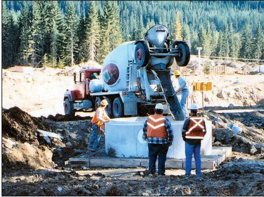
Figure 57.—Placement of a cast-in-place base slab for an inspection well.
