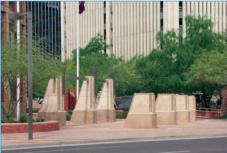
Figure 4-25: Group of engineered sculptured objects as a barrier.
