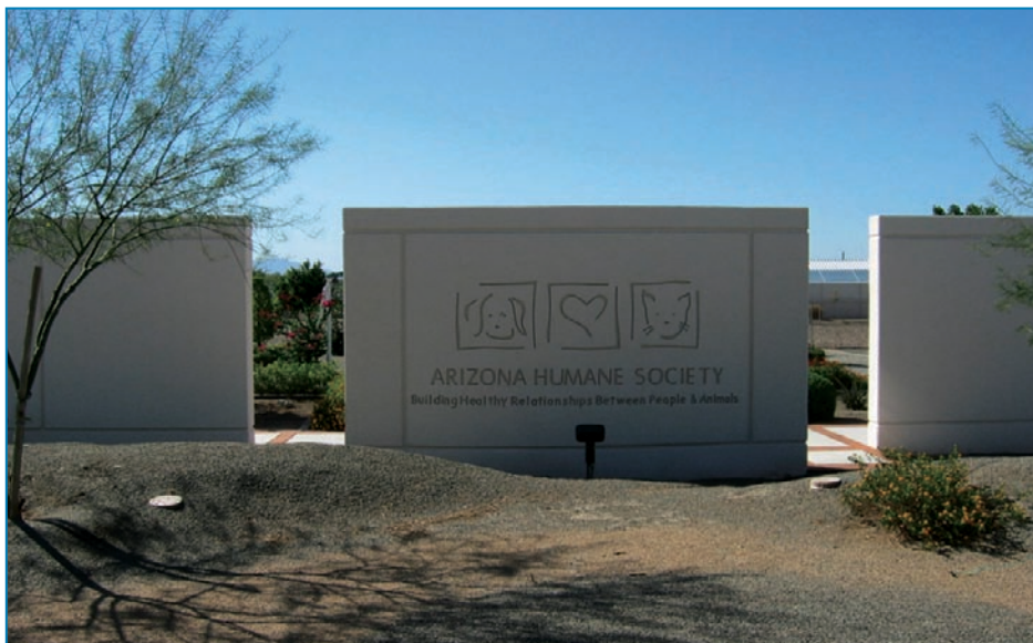
Figure 4-9: Reinforced wall barrier with artwork.
