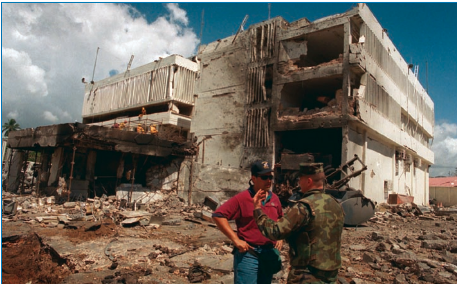
Figure 1-17: Damage to the U.S Embassy, Tanzania
