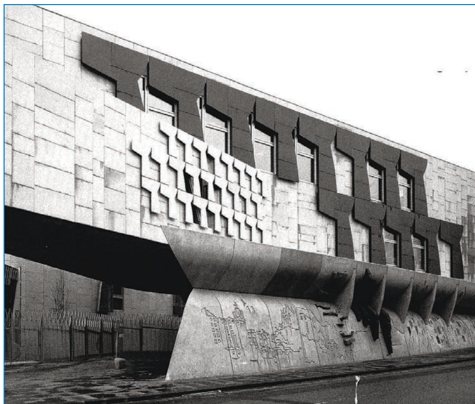
Figure 4-10: Reinforced concrete barrier wall with artwork at the Scottish Parliament, Edinburgh.
