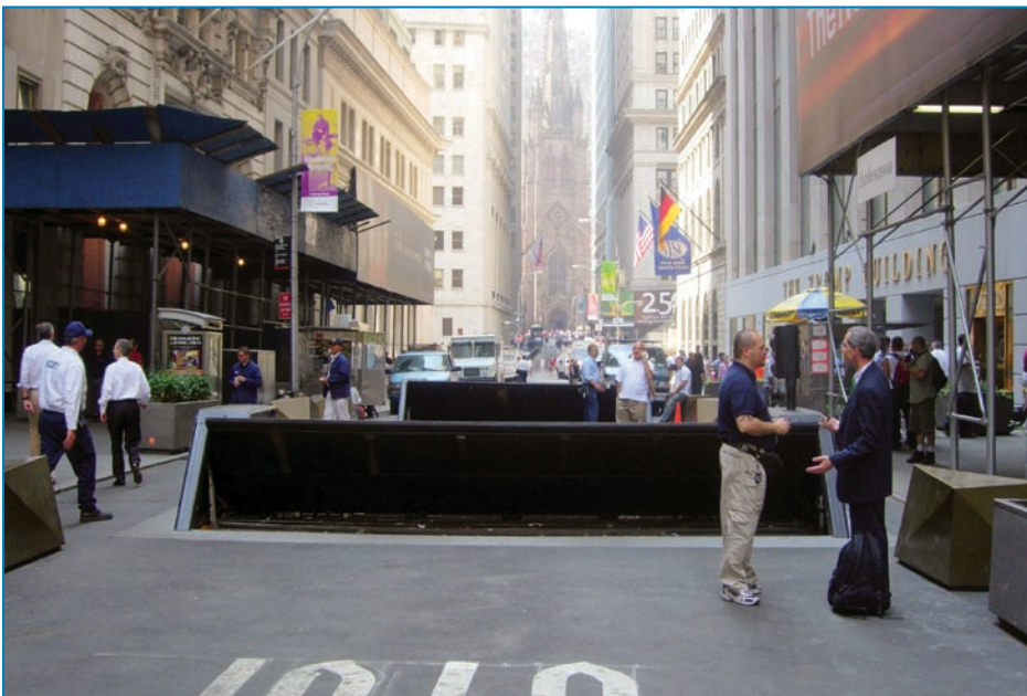
Figure 5-10: Sally port installation with two active barriers. Note NOGO barriers at the sides (see Section 4.6.1).
