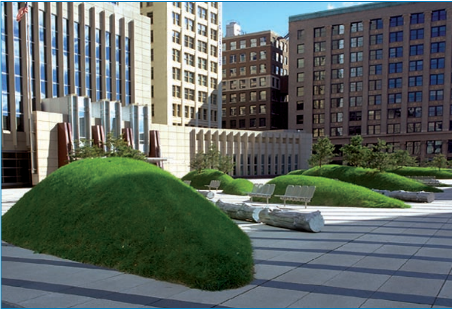
Figure 6-21: Minneapolis Courthouse plaza with planted berms, representing historic Minnesota “drumlins.” They also act as barriers to a vehicular attack, as a second layer of defense, creating stand-off.
