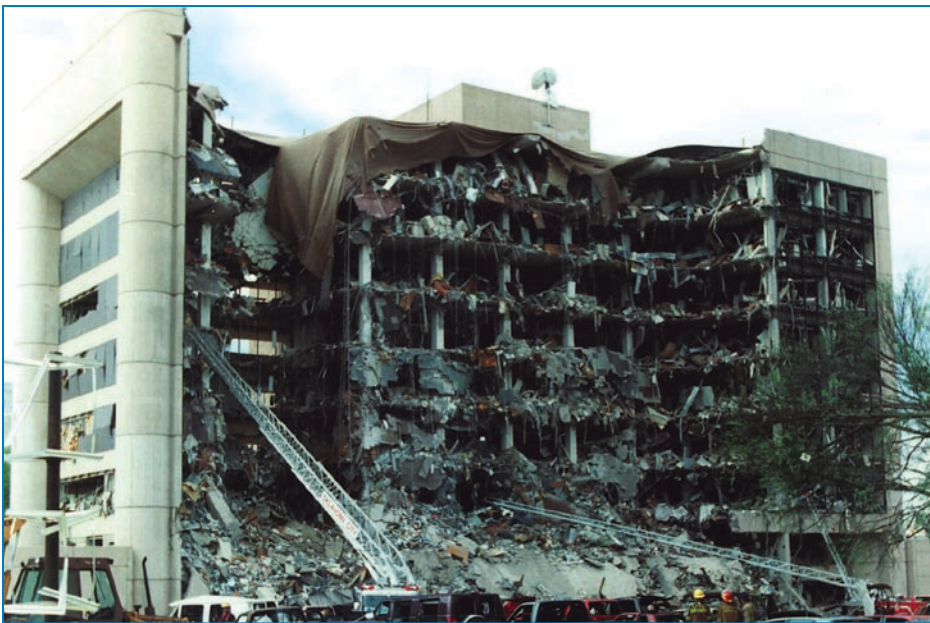
Figure 1-3: The Murrah Federal Building, Oklahoma City 1995.
