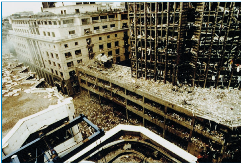
Figure 1-10: Damage to surrounding buildings SOURCE: © CORBIS
