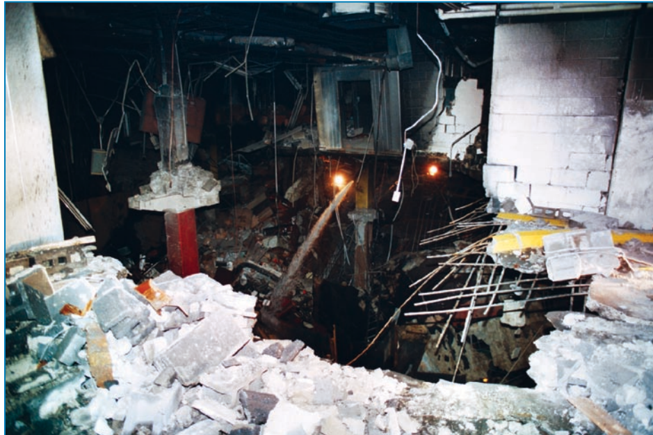
Figure 1-9: Damage in WTC garage caused by the 1993 bomb attack.
