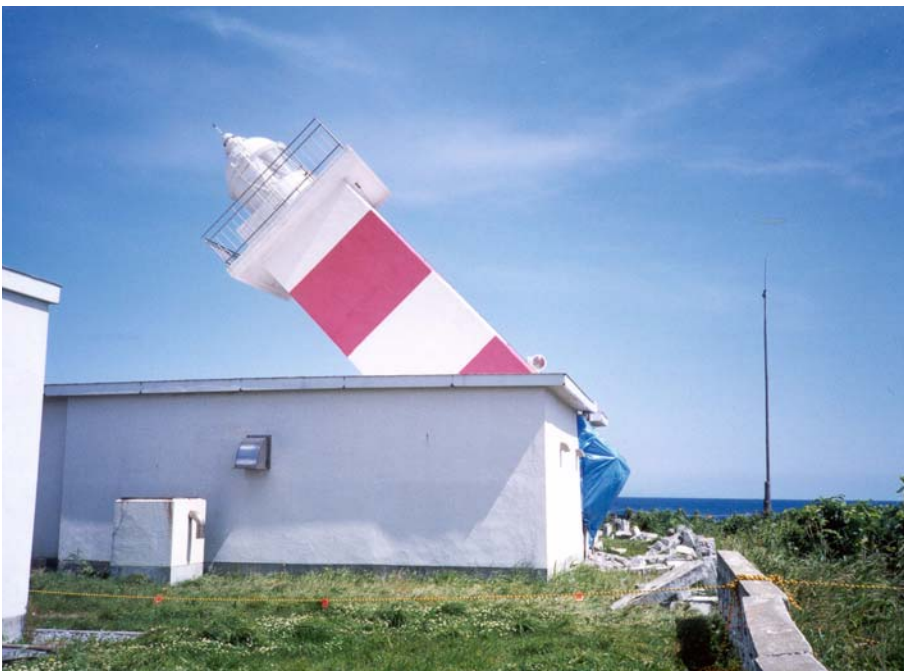
Figure 3-11 Overturned lighthouse at Aonae, Okushiri, from the tsunami following the 1993 Hokkaido-Nansei-Oki earthquake. (Photo courtesy of Yuji Ishiyama, Hokkaido University, Sapporo, Japan)
