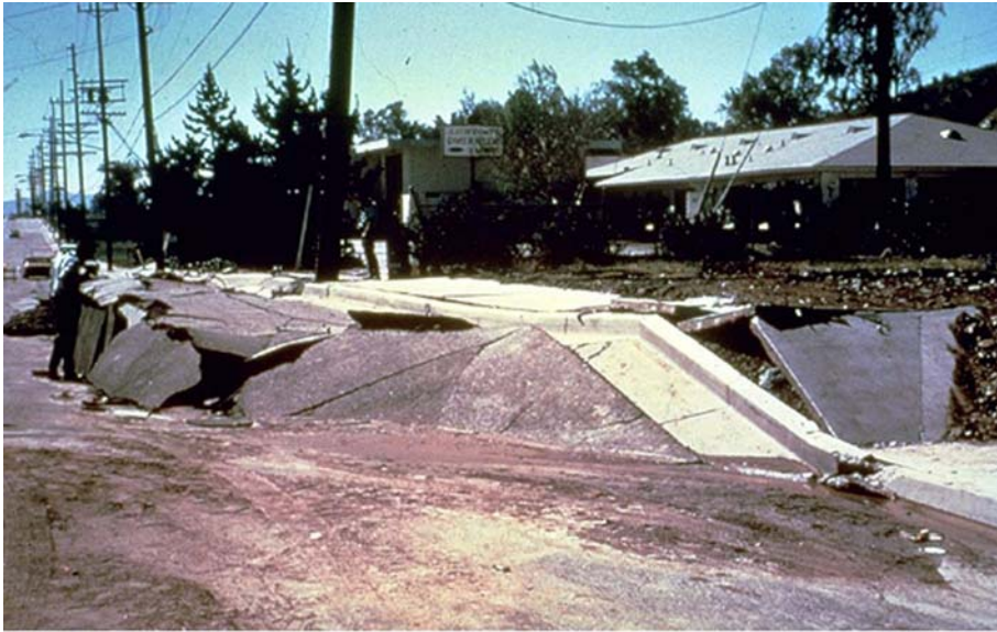
Figure 3-8 Example of surface fault rupture; 1971 San Fernando, California, earthquake (a thrust fault earthquake). (Photo courtesy of the Earthquake Engineering Research Institute.)
