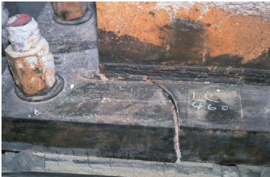
Figure 11-1 Fractured 4-inch-thick steel base plate, university building, Northridge, 1994. (photo courtesy of the Earthquake Engineering Research Institute)
