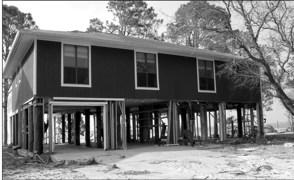
Figure 19. Structure elevated above BFE in AE zone showing successful response of breakaway walls
