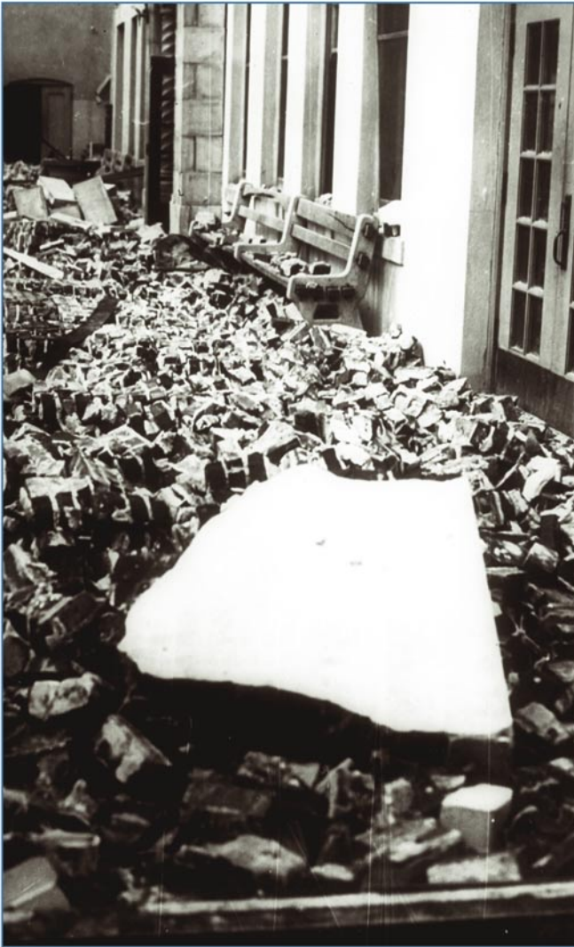
Figure 4-16 A dangerous passage way between two buildings, Polytechnic High School, Long Beach, CA, 1933
