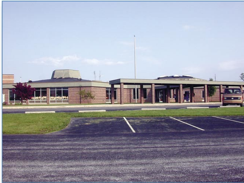
Figure 1-9 Elementary school, Fairfield, PA, 1980s
