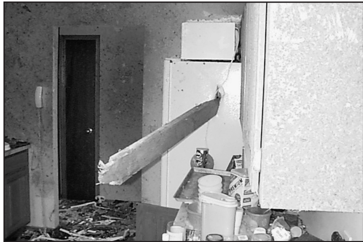
Figure 7-3. Refrigerator pierced by windborne missile (a 2x6 wood board), Moore, Oklahoma
