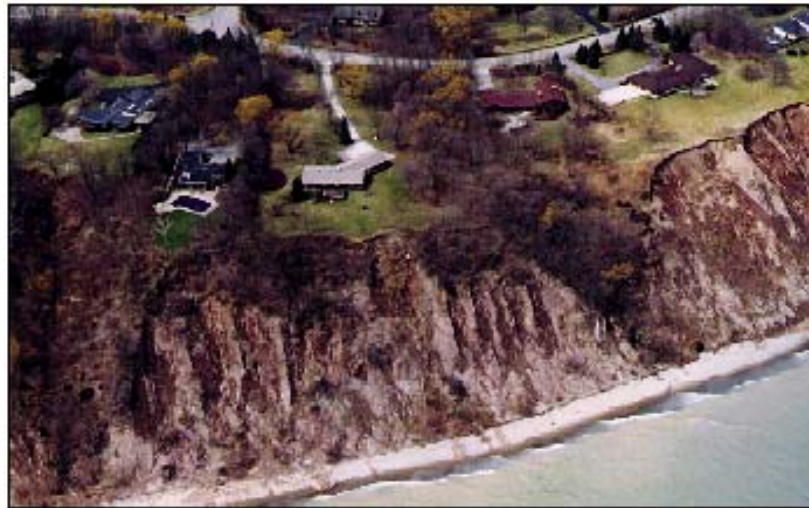
Figure 8-15. Residential buildings outside the floodplain threatened by long-term erosion along the Lake Michigan shoreline. Ozaukee County, WI (1996).
