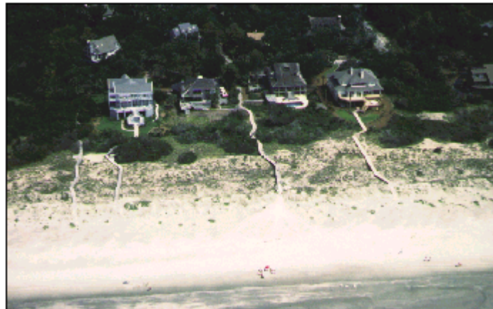
Figure 8-2. Example of coastal development well-suited to the land. Deep lots, generous setbacks, and avoidance of dune areas should afford protection against erosion and flood events for years to come.
