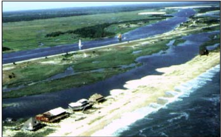
Figure 8-11. Not recommended. Construction along this narrow, low-lying area of St. Johns County, FL, is routinely subjected to coastal storm effects. The lots and buildings are landward of a previous State highway location, now abandoned.
