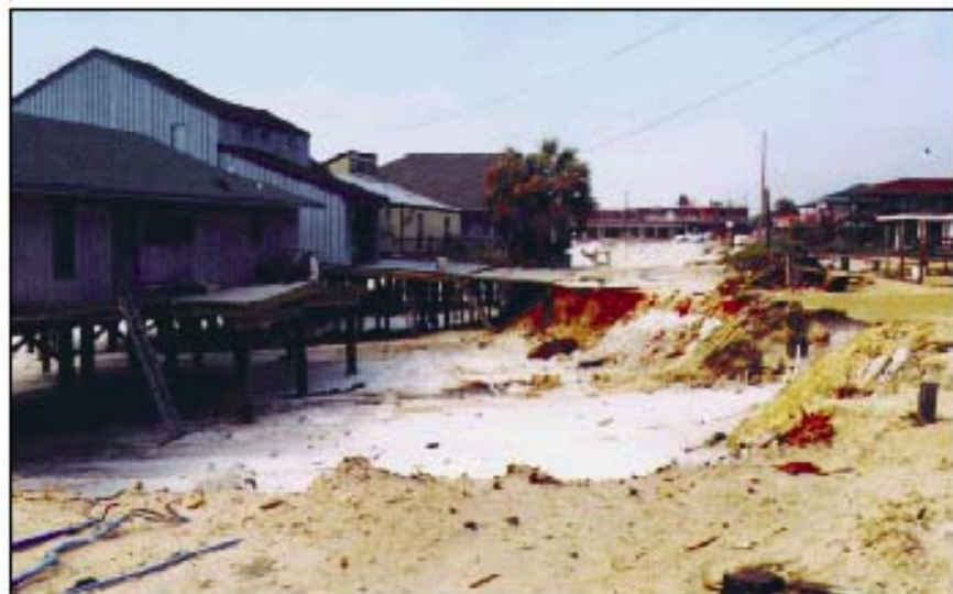
Figure 8-4. View along a washed-out, shore-parallel road in Bay County, FL, after Hurricane Opal. Homes to the left are standing on the beach and have lost upland access. Some homes to the right have also lost their roadway access.
