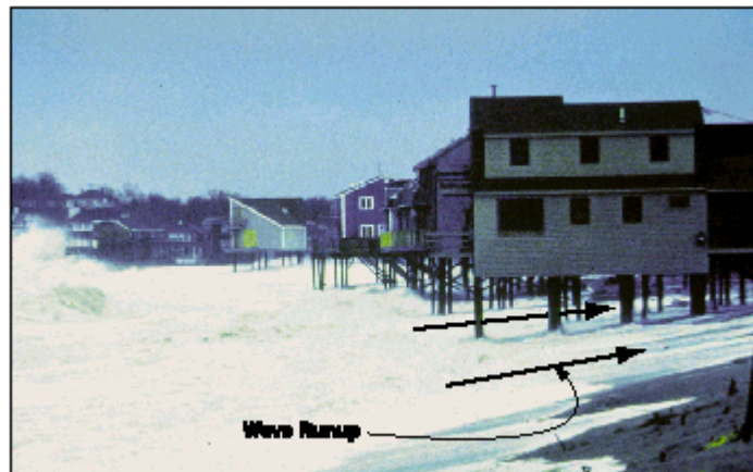
Figure 6-10. Wave runup beneath elevated buildings at Scituate, MA, during the December 1992 northeaster. Nine homes in the area were bought with public funds and demolished following the storm.
