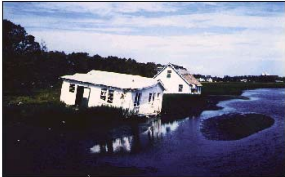
Figure 6-4. Hurricane Hugo (1989), Garden City, South Carolina. Intact houses were floated off their foundations and carried inland.
