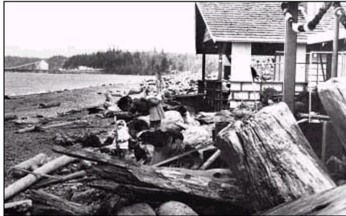
Figure 6-15. March 1975 storm. Drift logs driven into coastal houses at Sand Point, WA.
