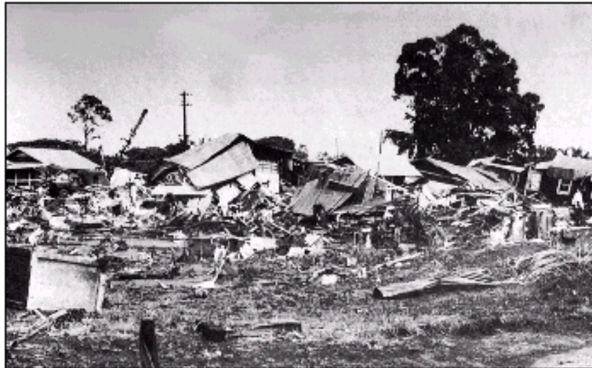
Figure 6-3. Hilo, Hawaii— damage from the 1960 tsunami
