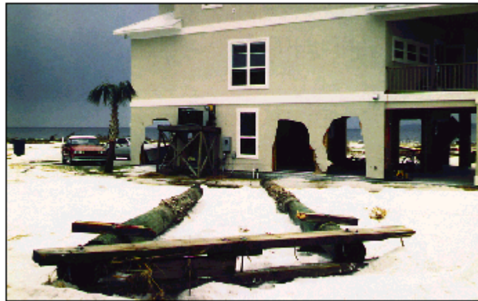
Figure 6-13. Hurricane Opal (1995). Pier pilings were carried over 2 miles by storm surge and waves before they came to rest against this elevated house in Pensacola Beach, Florida.
