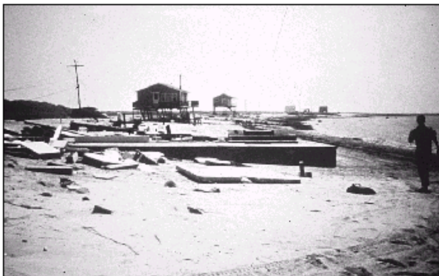
Figure 1-2. Hurricane Bob (1991) destroyed 29 homes along this reach of Mattapoissett, MA.
