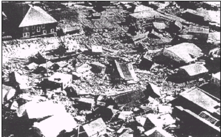
Figure 1-13. 1964 Good Friday earthquake. Damage in Kodiak City, Alaska, caused by the tsunami of the 1964 Alaskan earthquake.
