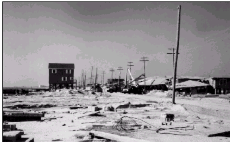
Figure 1-4. Hurricane Hugo (1989), Garden City Beach, SC. House on pilings survived while others did not.
