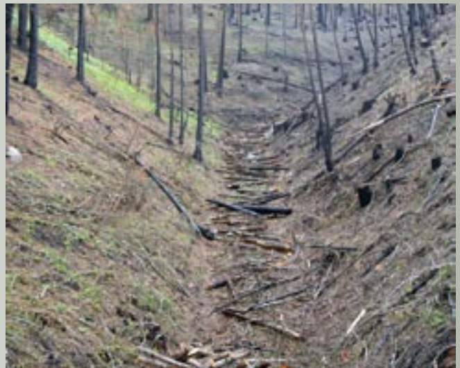
The same area has been seeded with slender wheatgrass, dead trees have been harvested, and logs have been placed in the draw to slow water movement.
