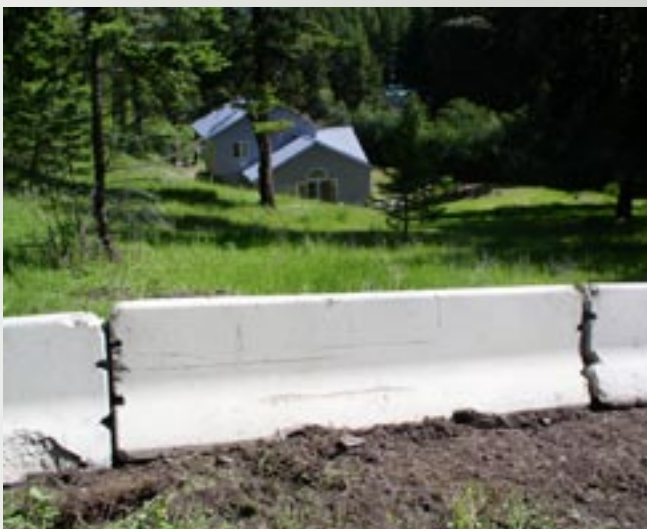
Concrete barriers have been placed on the hill above this home to divert potential water and debris flows.
