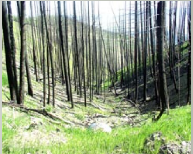
The private roads and culverts were protected and armored to allow more water and debris to pass through and over the road during high flow events.
