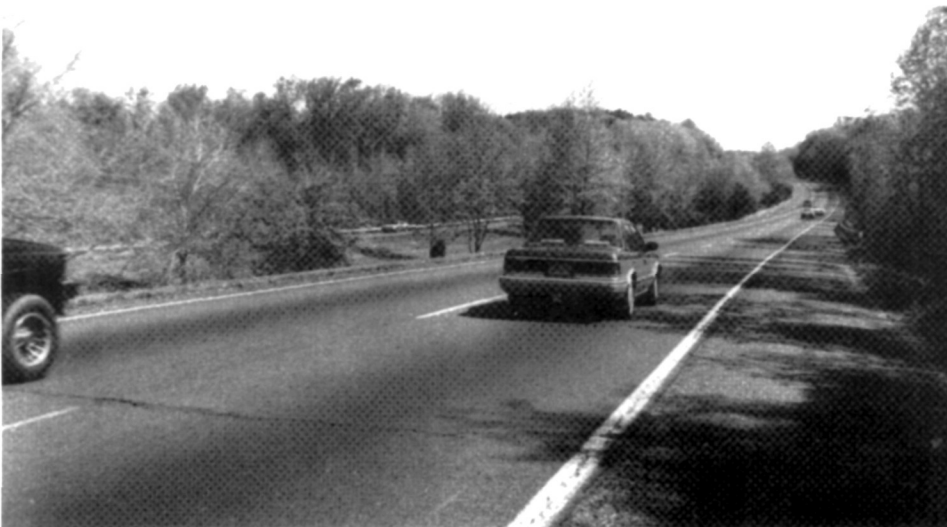
The Baltimore-Washington Parkway in Anne Arundel and Prince George's counties, Maryland, was constructed between 1942 and 1954 as a component of a national parkway system. (Sara Amy Leach, April, 1988)
