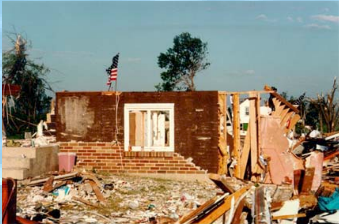
Senior citizen's home destroyed by tornado. FEMA photo by Brian Hvinden
