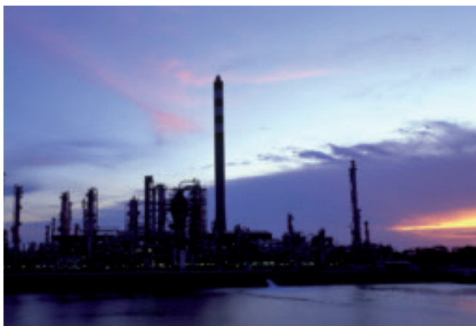
The Long Residue Catalytic Cracking Unit (LRCCU) on Pulau Bukom
