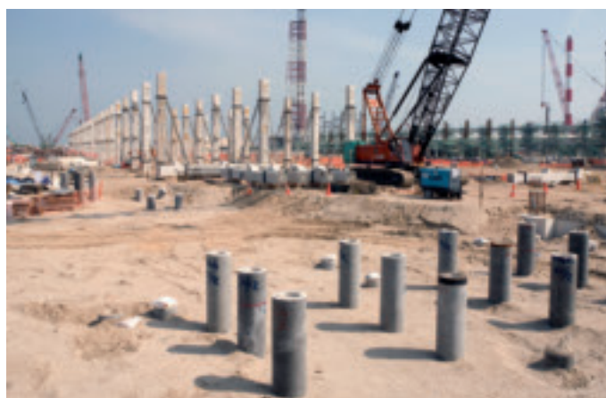
Construction at Bukom Island
