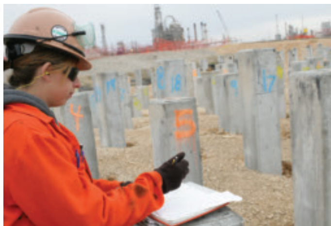
Construction at Port Arthur
