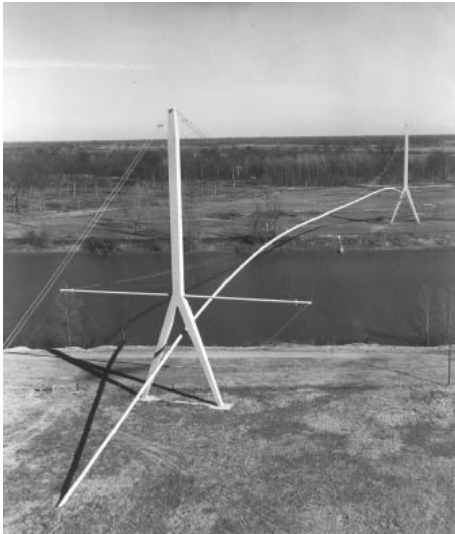
An overhead pipeline crossing on the White River near Newport, Arkansas.
