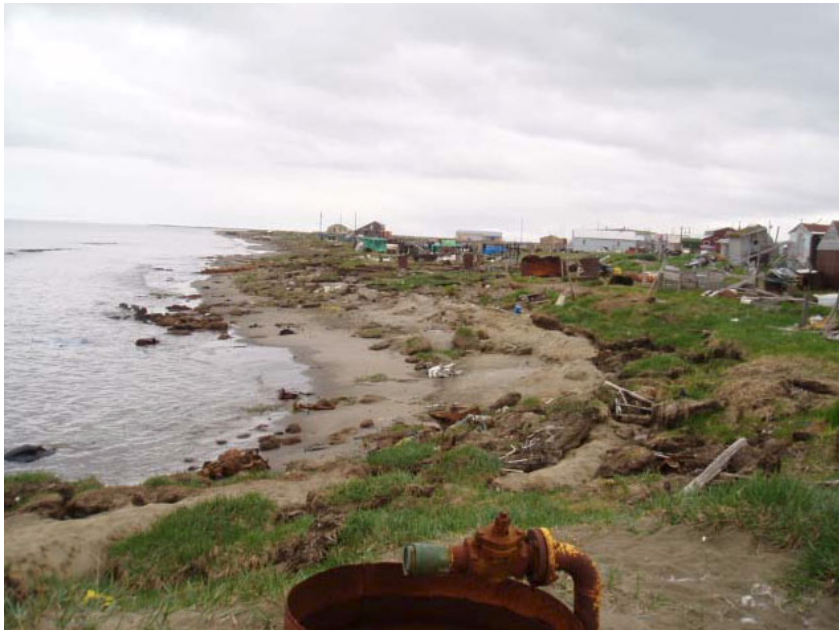
Center of town looking east
