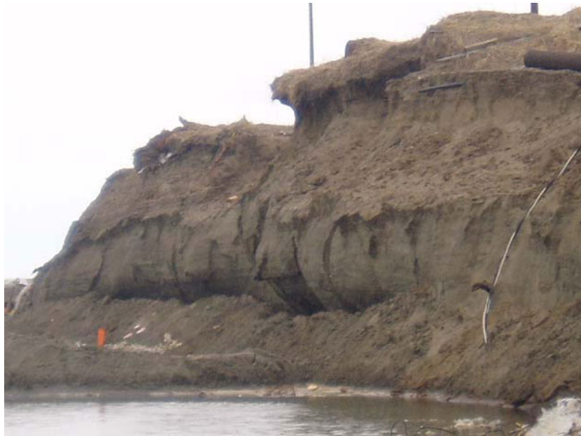
West end permafrost exposed and melting
