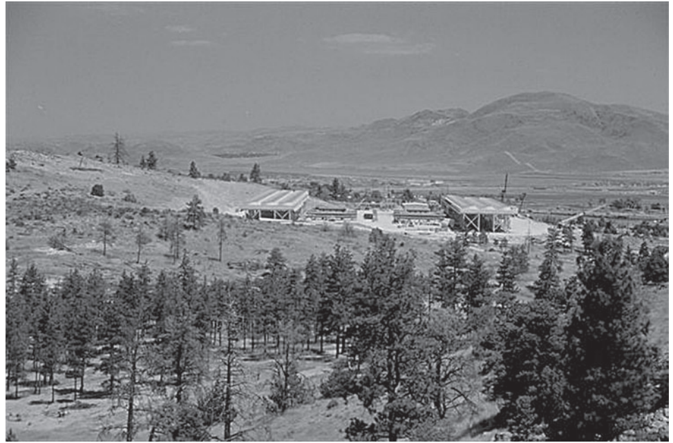
Figure 2: Geothermal Power Plant near Reno, Nevada
