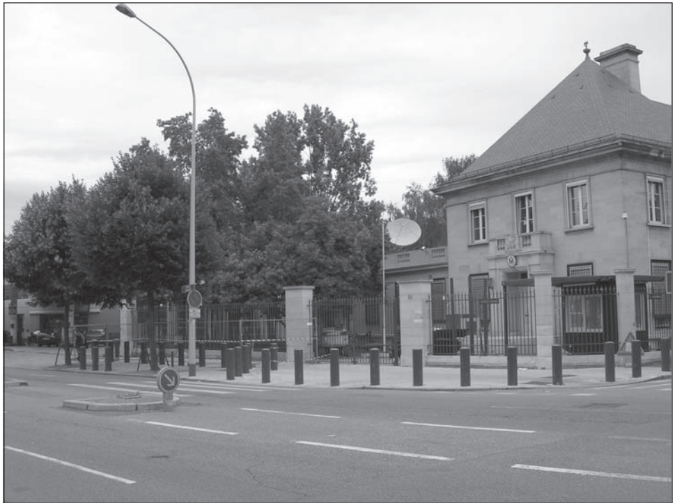
Figure 5: A Post with Insufficient Setback
