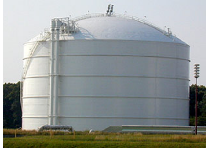
LNG Storage Tank at Cove Point, MD
