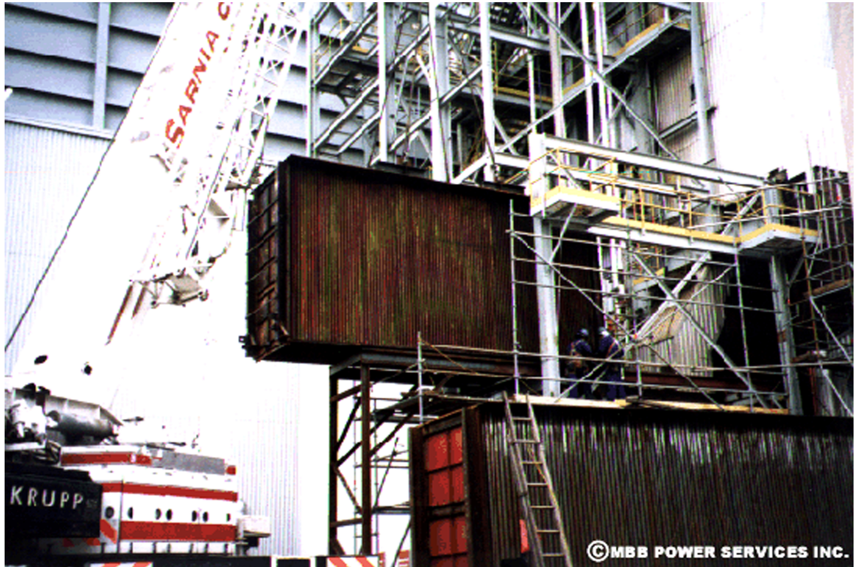
Removal and installation of airheater
