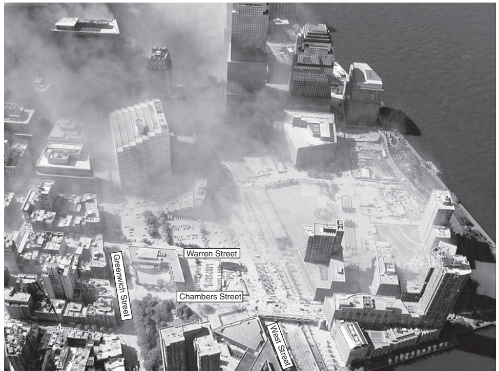
Figure 2: Collapsed WTC Towers on September 11, 2001
