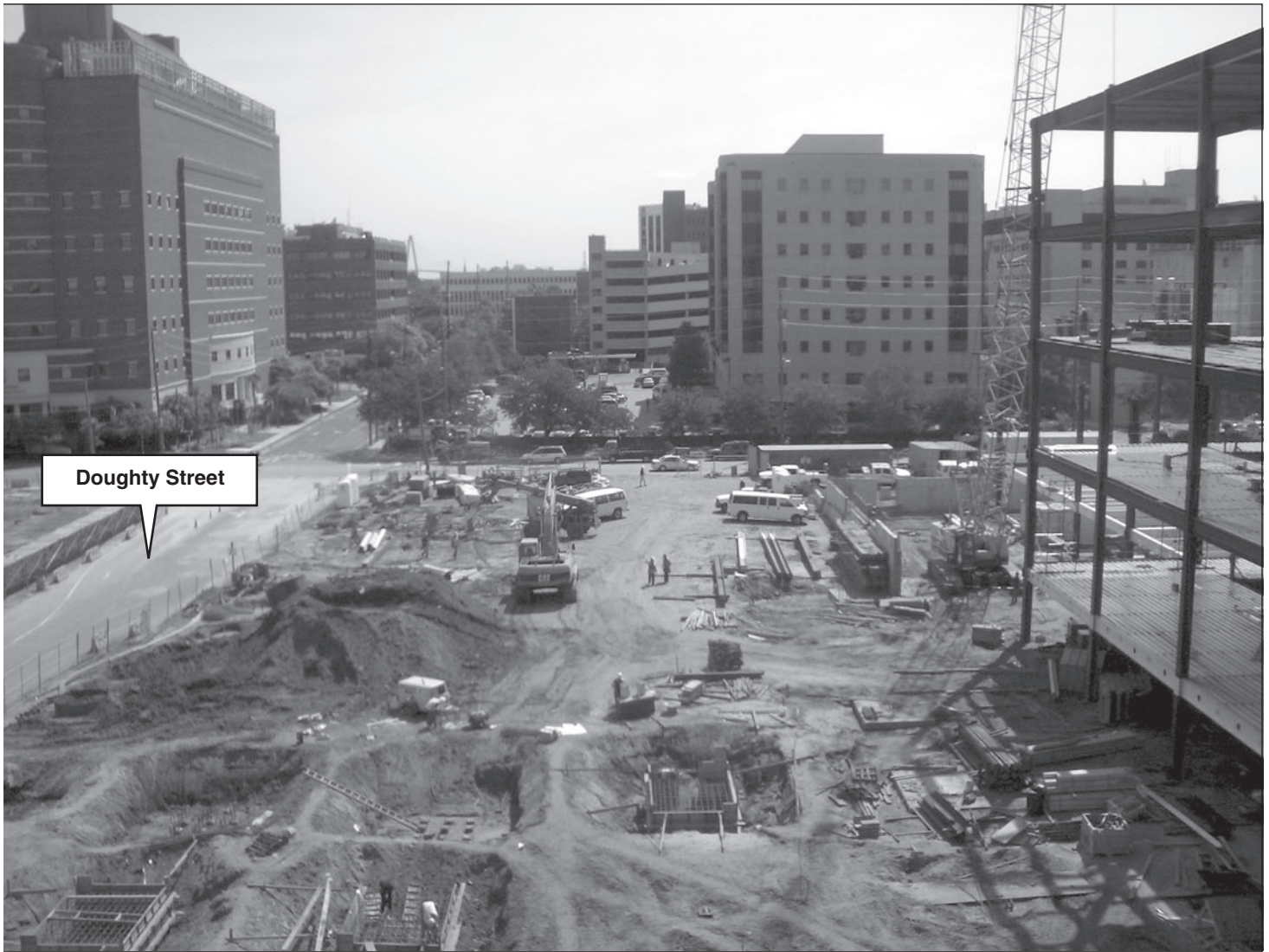
Figure 7: Construction of Phase I of MUSC's Project, July 2005
