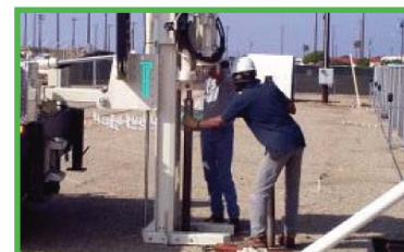
FIGURE 3. In Situ Bioremediation of MTBE in Groundwater Using Propane Oxidizing Bacteria, Envirogen, Inc.
